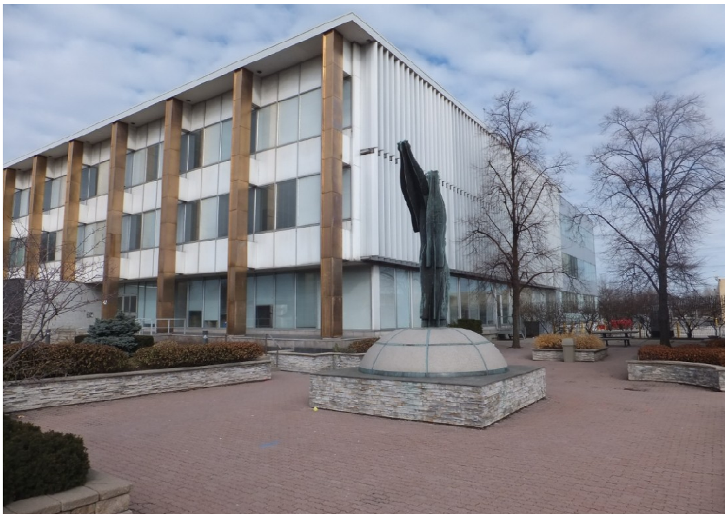
Above: principal (south) façade of the Coca-Cola Office Building Below: "Coca-Cola" sculpture in the courtyard adjoining the office building (left) (Heritage Preservation Services, March 2013)
