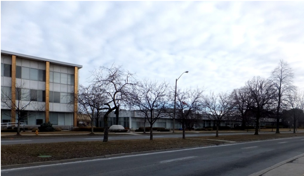
11. Current Photographs: looking west (above) and east (below) on Overlea Boulevard and showing the Coca-Cola Building and the adjoining bottling plant (Heritage Preservation Services, March 2013)
