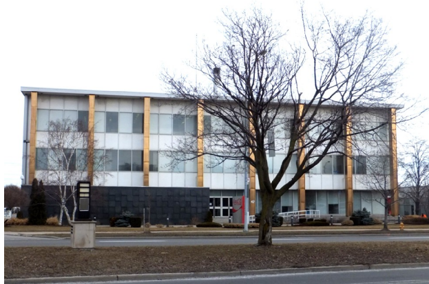
Principal (south) façade of the Coca-Cola Building (Heritage Preservation Services, March 2013)
