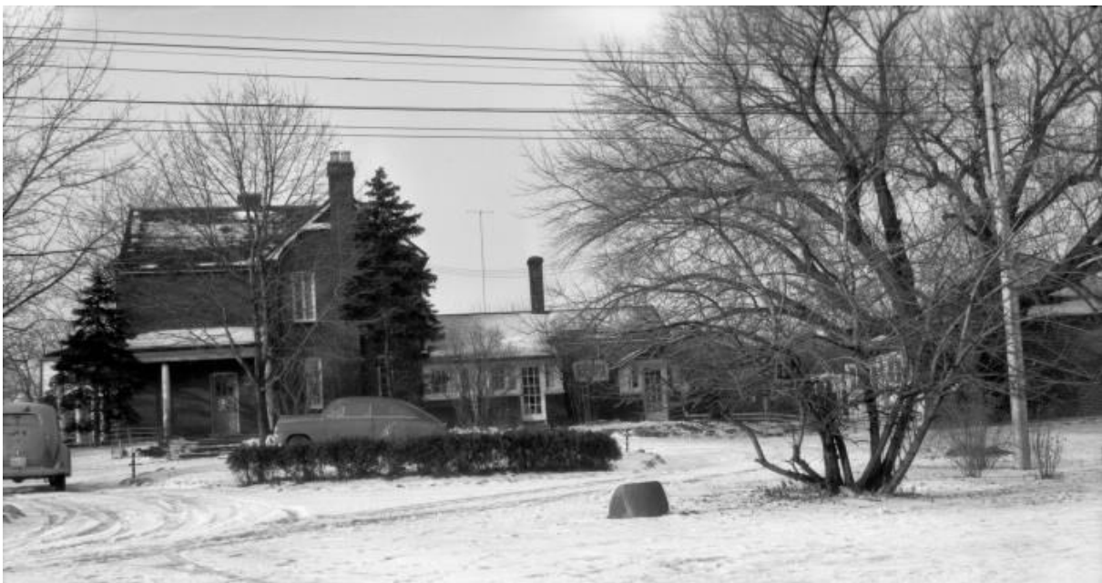
22. Archival Photographs, 262 Bessborough Drive, 1955 : showing the north wing of the Thomas G. Elgie House on the right before it was altered in 1990 (Toronto Reference Library, Item 3400)
