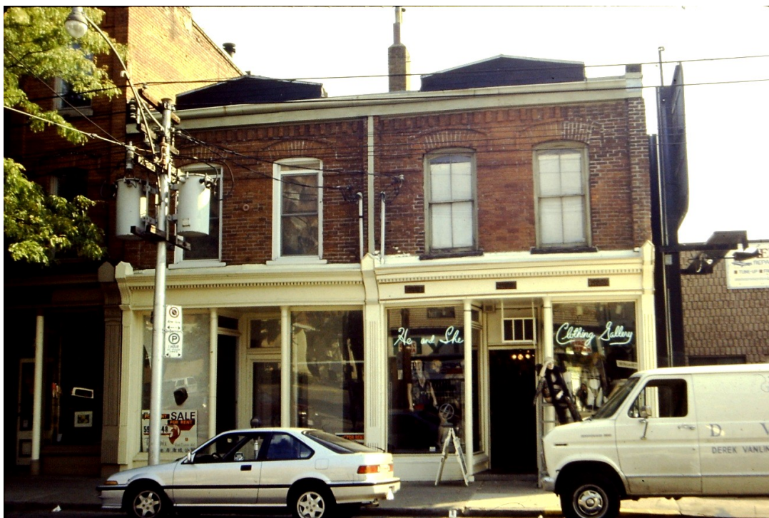
12. Archival Photograph, 263-265 Queen Street East, 1993: showing the storefronts with recessed entrances and the decorative brickwork on the second-storey openings and beneath the roofline (Toronto Historical Board)
