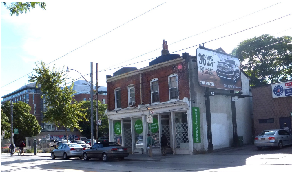
Showing the principal (north) façades (above) and the context of the Christina Lauder Buildings on Queen Street East (below) (Heritage Preservation Services, September 2013)
