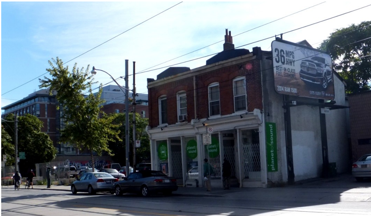
13. Current Photographs, 263-265 Queen Street East, September 2013: showing the gable roofline and the exposed west elevation (Heritage Preservation Services)
