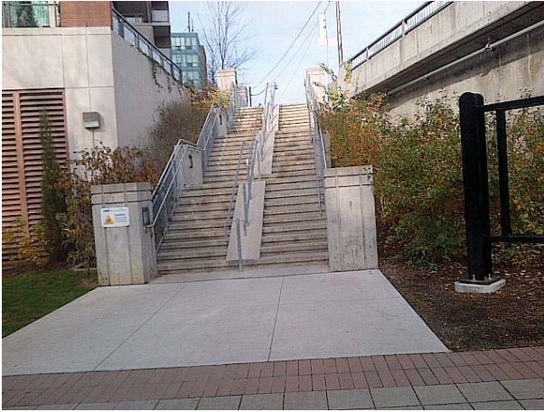
Left: Stairs at Merton and Mt. Pleasant Rd.
