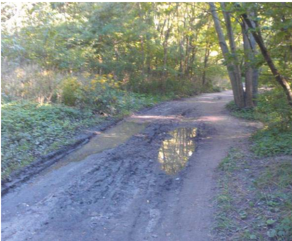
Left: Poorly drained trail at David Balfour park
