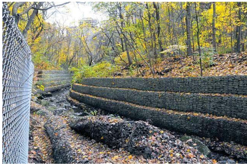
Left: Mt. Pleasant Cemetery, plane tree Right: Vale of Avoca. Wire mesh Gabion cages reinforce the banks of Yellow Creek
