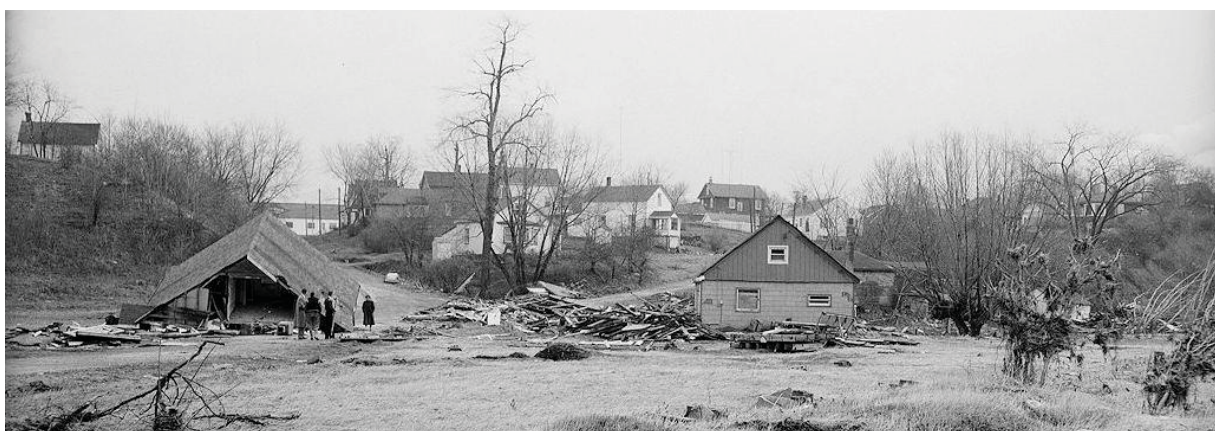
Flood damage at Eglinton Flats, aftermath of Hurricane Hazel. 1954. Located 1 km. north of Humber Beltline loop
