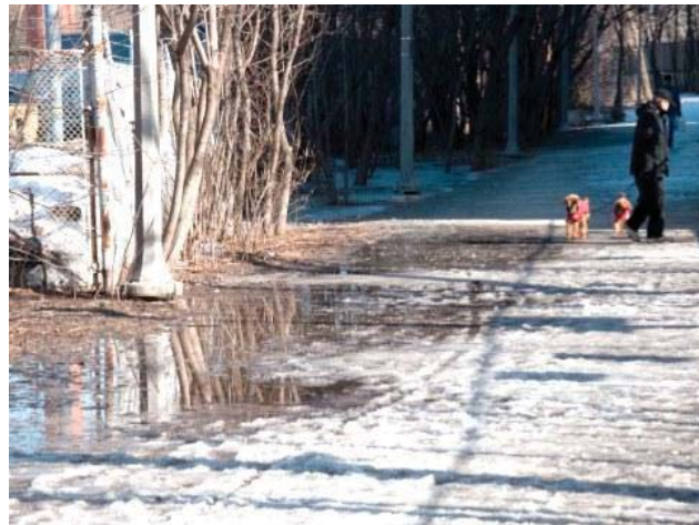
Right: Flooding on trail east of Lascelles Blvd.
