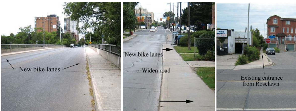
Left: Elm Ridge Dr. bridge over Allen Road
