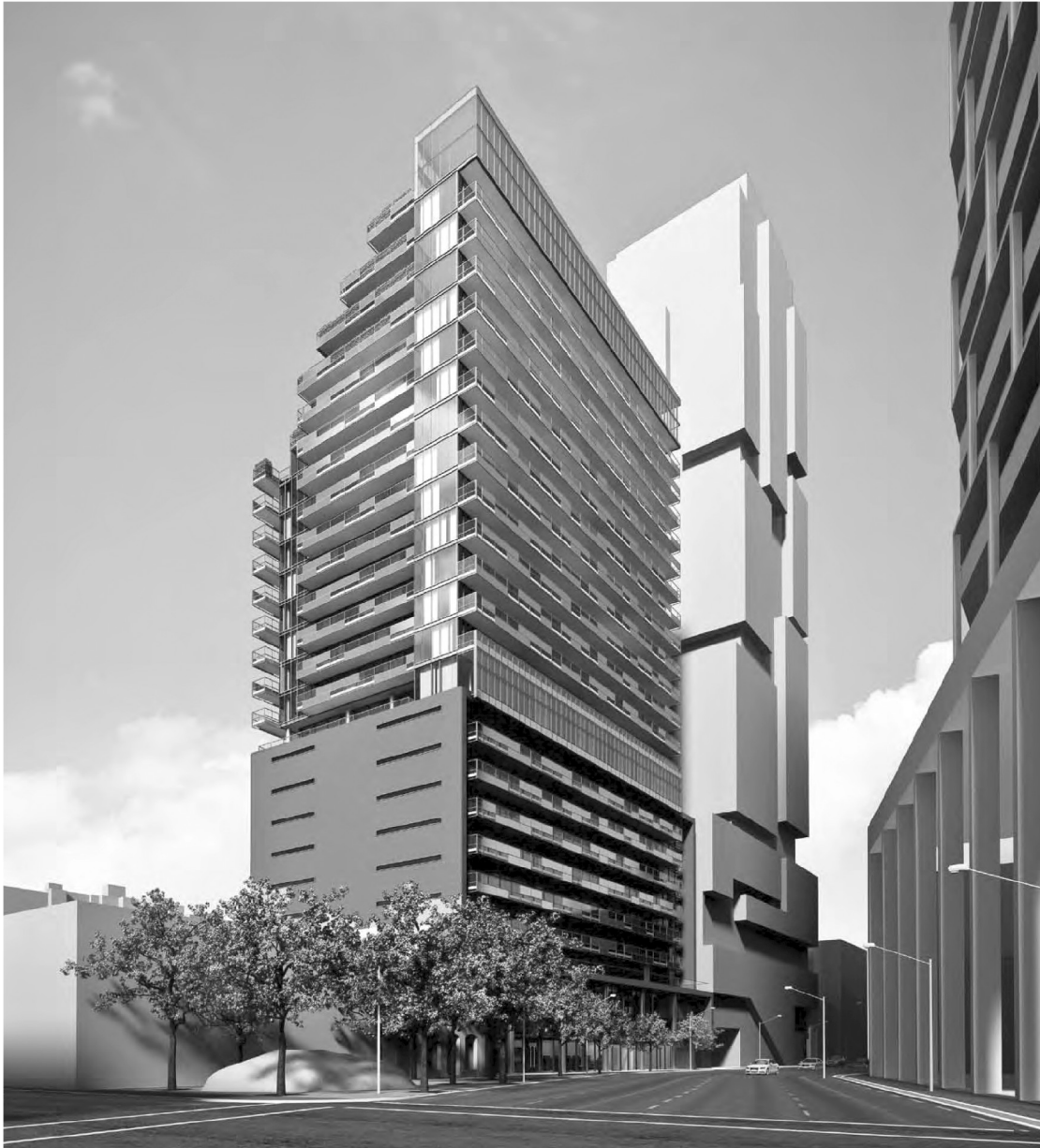
Looking east along Richmond Street West
