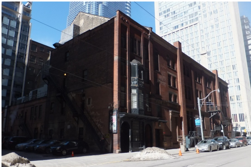
29. Current Photograph, Massey Hall : showing the east elevation on Victoria Street (right) and the rear (south) wall (left) with the two-storey Annex on the extreme left (Heritage Preservation Services, 2013)
