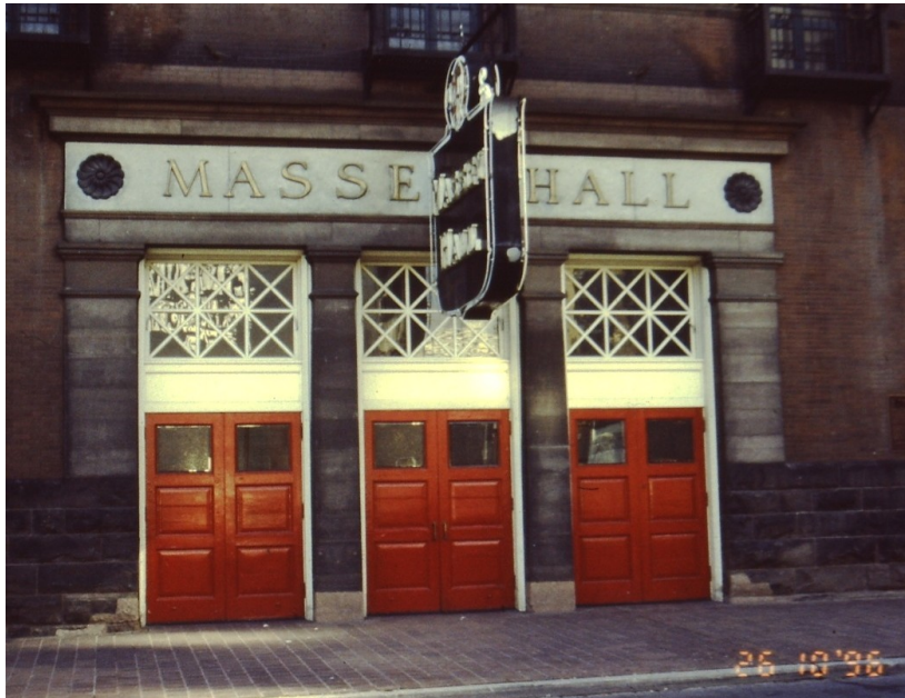
26. Photograph, Massey Hall, 1996 : showing the north entrance and signage (Toronto Historical Board)
