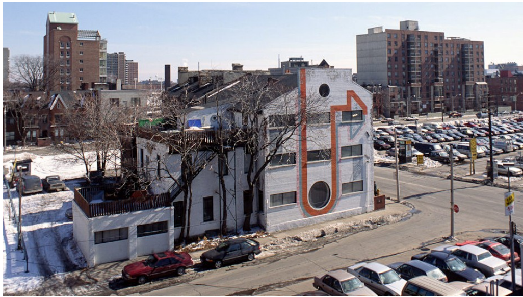
17. Archival Photograph, Shuter and Dalhousie Streets, 1970s : showing the rear (north) ends of the Edward Cooper Houses on the left, with the neighbouring Gillespie Houses (right) (City of Toronto Archives, Series 1465, Item 10)
