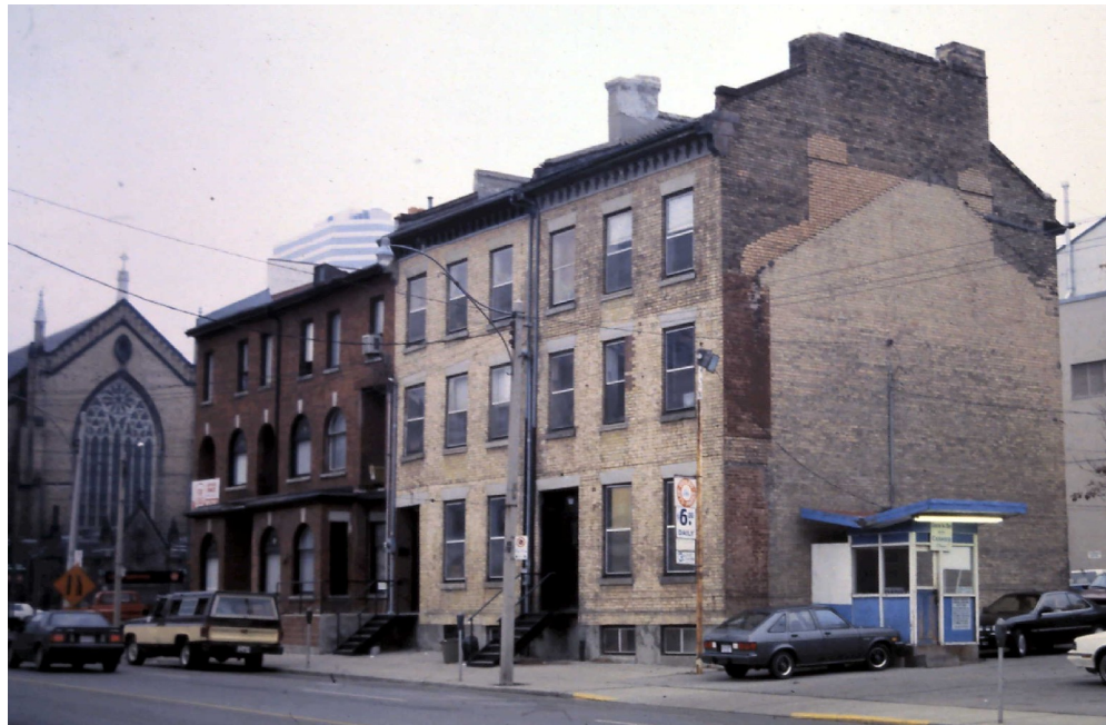
18. Archival Photograph, 64-70 Shuter Street, 1970s : showing the Edward Cooper Houses with the imprint of the former house form building at 72 Shuter Street on the east elevation of 70 Shuter (Toronto Historical Board)
