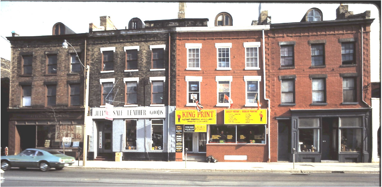
15. Archival Photograph, Hughes Terrace, 319-325 King Street West, 1973 : showing mid 19th century row houses designed by architect John Tully (Toronto Historical Board, 1973)
