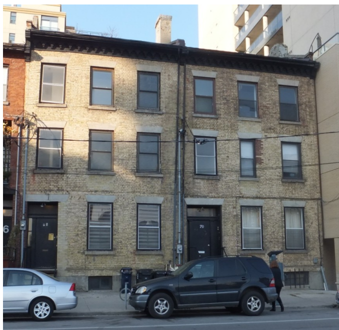
Cover and above: principal or south facades of the Edward Cooper Houses at 68 and 70 Shuter Street (Heritage Preservation Services)
