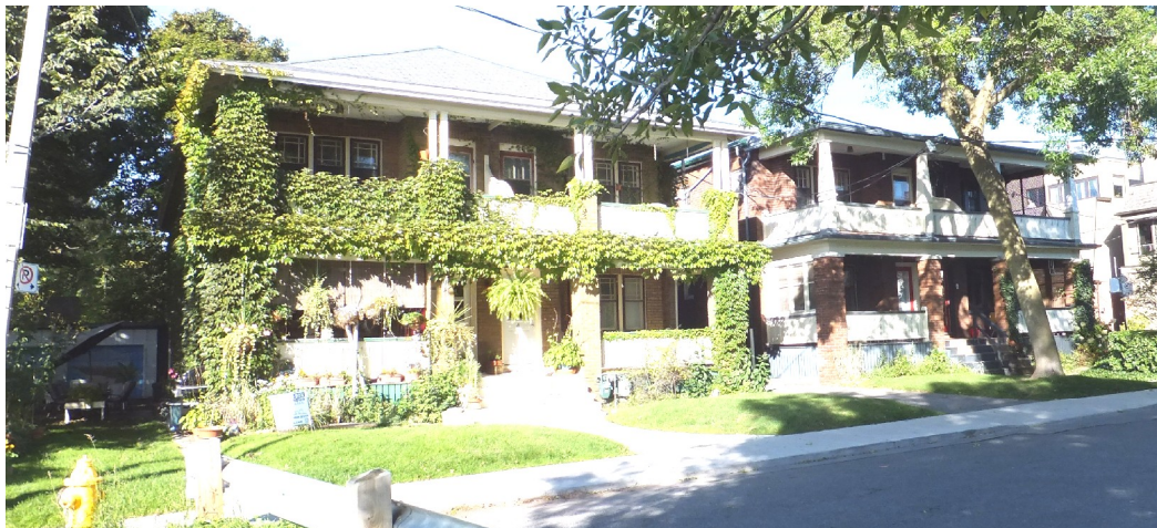
13. Current Photographs, 2-8 Wineva Avenue: showing the Fourplexes at 2-4 Wineva (top, left) and 6-8 Wineva (top, right), south of Hubbard Boulevard (centre) and from the waterfront (below) (Heritage Preservation Services)
