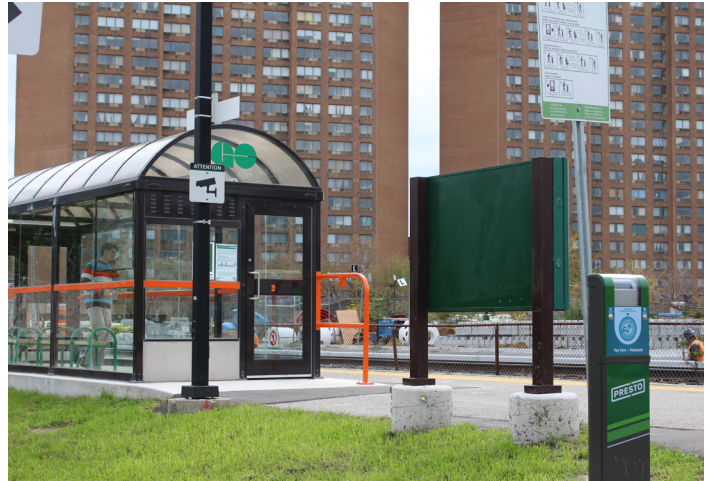
Bloor GO Station along the Georgetown Rail Corridor
