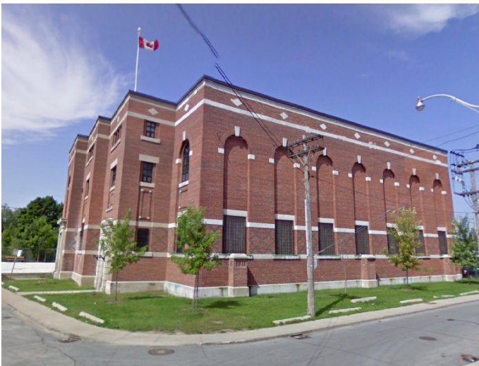
A. Toronto Hydro-Electric System Substation
