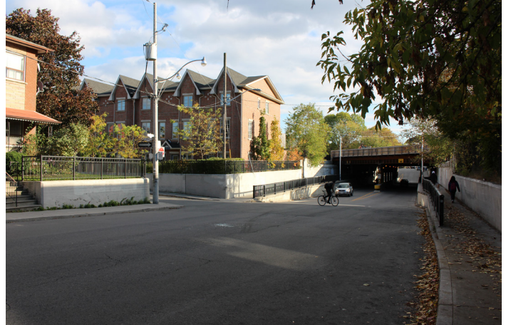
Florence and Brock intersection would benefit from installation of a traffic light and changes to the design of the railing.
