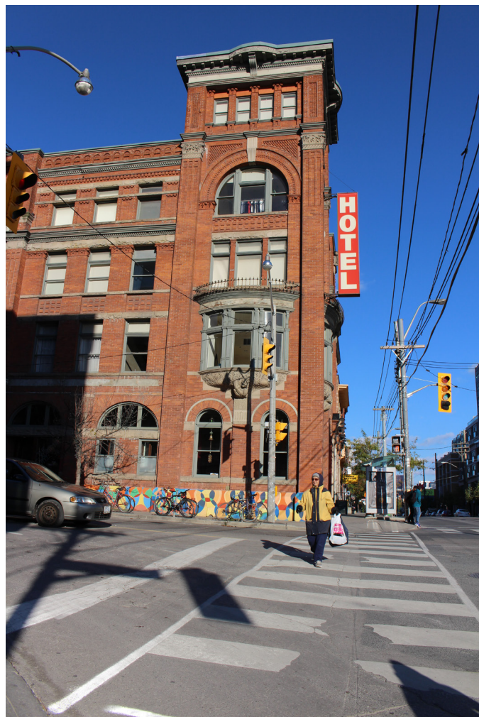
Pedestrian crosswalks should be installed at intersections.
