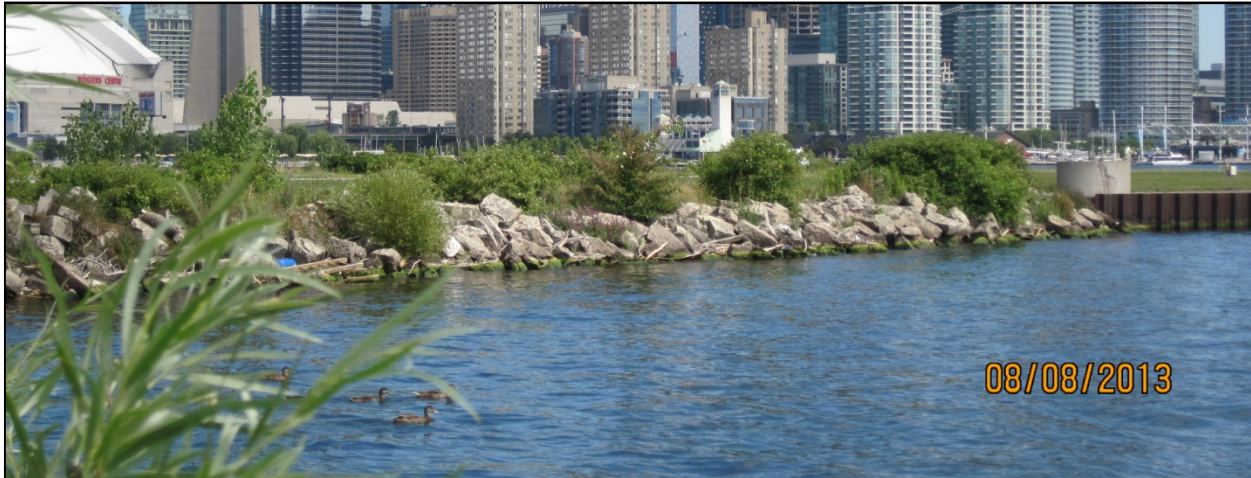
Figure 3-3 The Southeastern Revetment (Face A)
