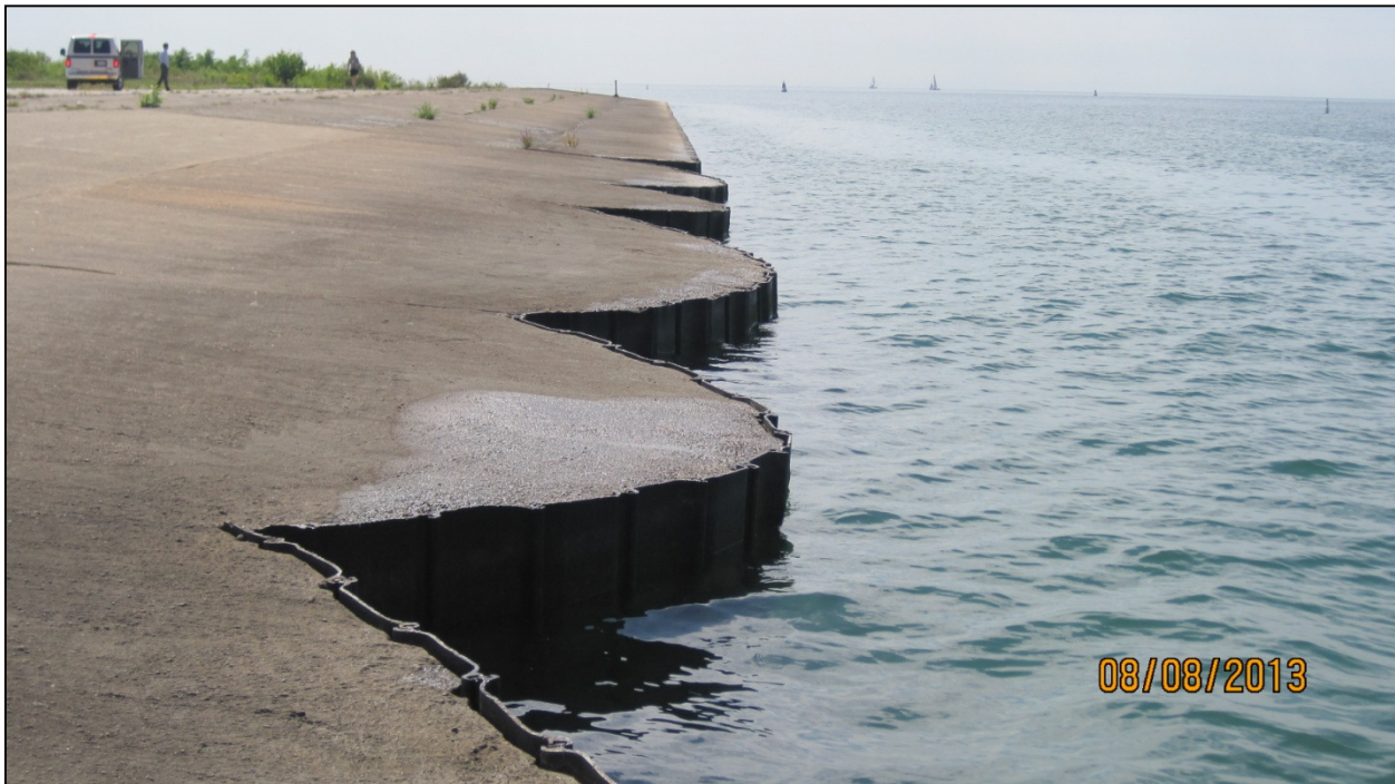
Figure 3-8 View South of the Northeastern Cellular Quay
