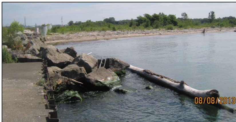
Figure 2-2 South of the Western End of the BBTCA Runway, Riprap and Floating Woody Debris Forms Structural Cover for Fish Species and Protection from Predators
