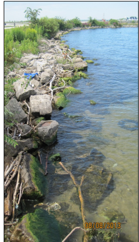
Figure 3-5 Sand Accumulation at the Eastern End of the Northeastern Revetment
