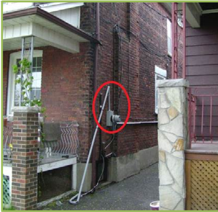
Figure 14: Example of Mast Damage
