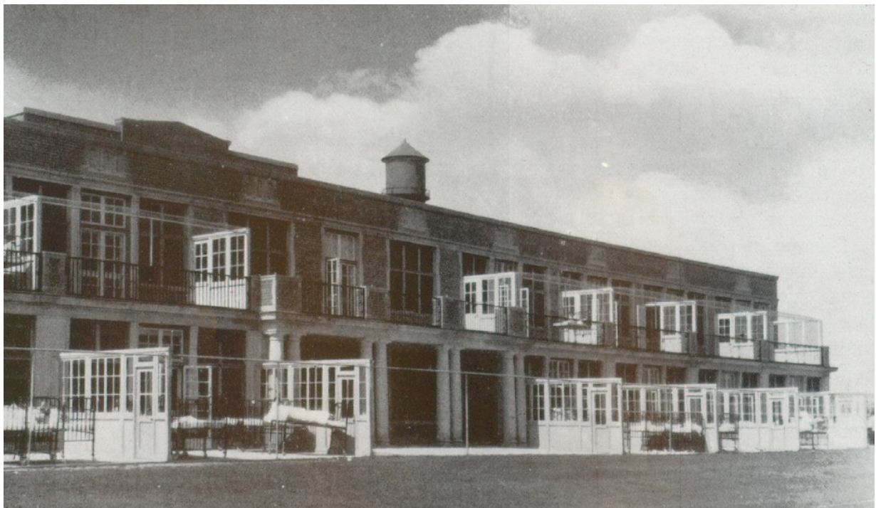
Below: South façade of the former Sick Children's Hospital (County Branch) Thistletown, now the Thistletown Regional Centre for Children and Adolescents (Construction Journal, June 1929)
