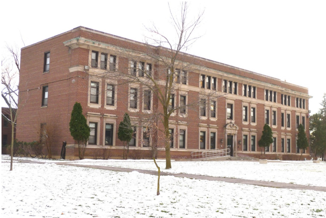
Above: principal (north) façade of the former Sick Children's Hospital (County Branch) Thistletown, now the Thistletown Regional Centre for Children (HPS 2013)
