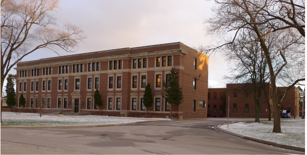
5. North Façade with rear side of South Wing (Heritage Preservation Services, December 2013)
