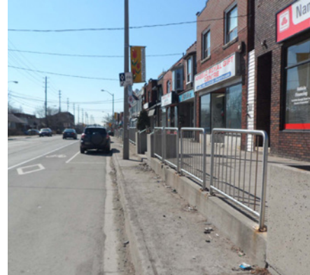
Existing conditions along Royal York Rd.
