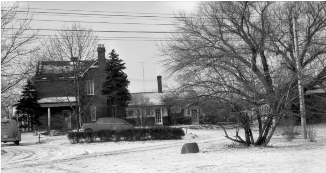
Archival photo showing east view of the Thomas G. Elgie House from Bessborough Drive including addition on north side of house Source: Toronto Public Library
