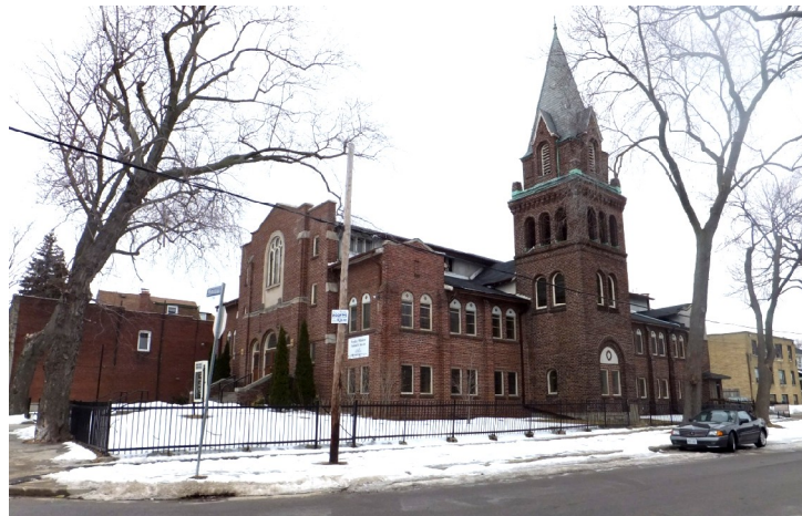
2 Station Road : showing the rear north wall (top), east elevation along Station Road (middle) and the south elevation (Heritage Preservation Services, February 2013)
