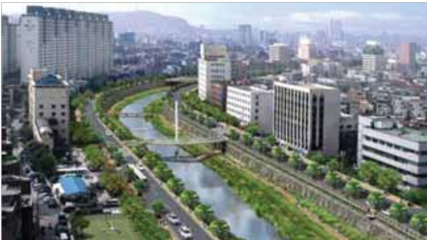
The Cheonggyecheon Expressway contributed to declining property values and population loss in Seoul's downtown before it was replaced by a linear park.
