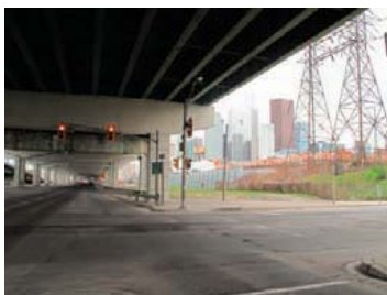
The elevated structure is a perceived barrier to the waterfront – pedestrians can walk under it, but public realm conditions are harsh.
