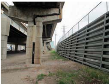
The elevated structure is a barrier.
