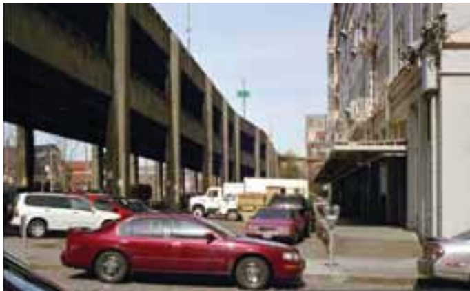
Existing condition under the Viaduct.
