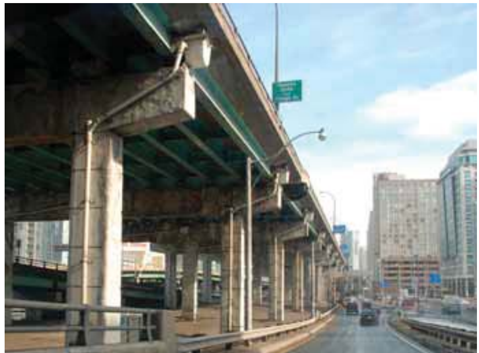
Gardiner Expressway in downtown Toronto.
