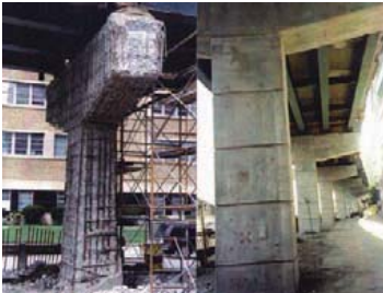
Some corroded concrete columns have been repaired.
