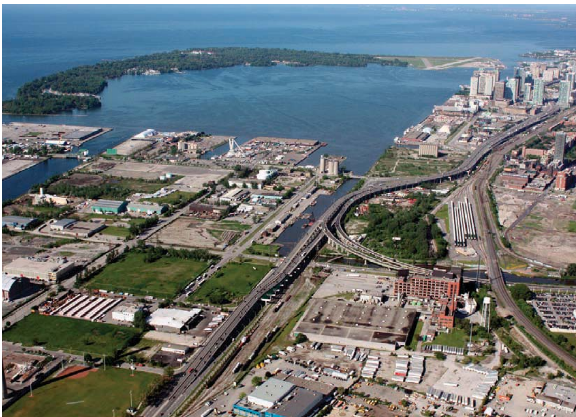
View of Gardiner Expressway and the Inner Harbour from the east.
