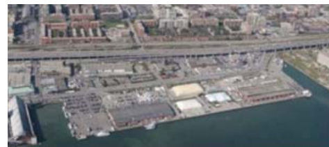
East Bayfront Precinct – Existing.
