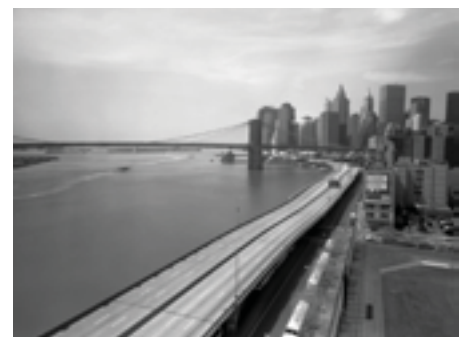
Views of F.D.R. along the East River facing south towards Lower Manhattan.
