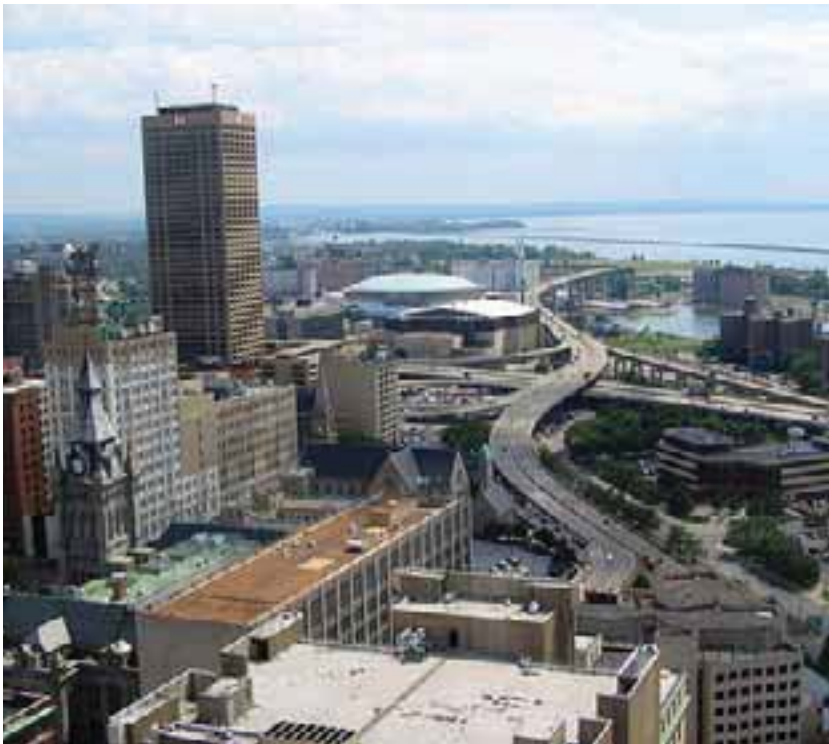
View of Skyway facing south.
