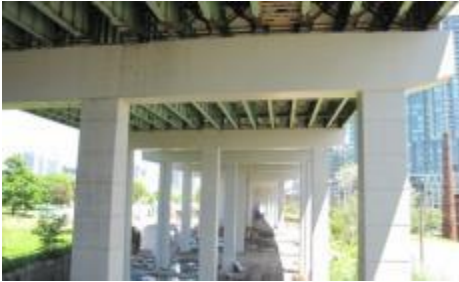
KEY IDEA – Rehabilitated Infrastructure: Rehabilitating the existing columns and girders of the Gardiner East. (Gardiner Expressway at Fort York).
