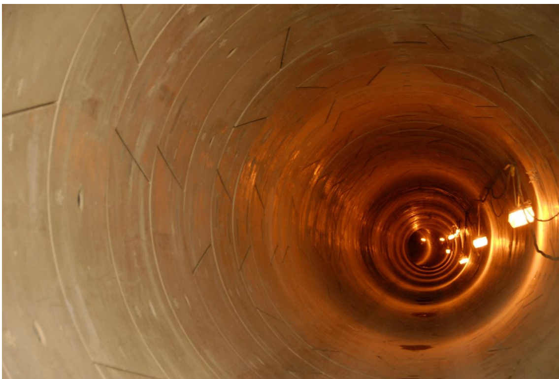
Figure 3 Photograph of New Permanent By-pass Tunnel
