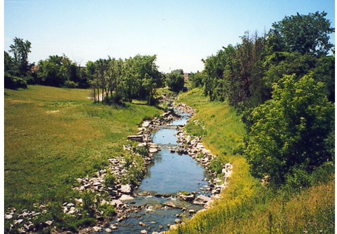
Fig. 21: Existing Photo - East Highland Creek
