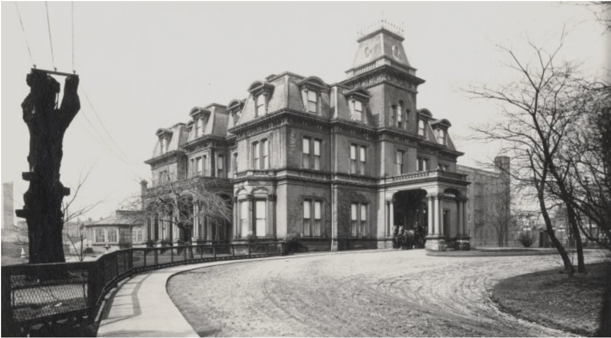
12. Archival Photograph, Government House (completed 1870), King and Simcoe Streets, 1912 : the Lieutenant Governor of Ontario's official residence introduced the Second Empire style to Toronto (Toronto Reference Library, Item 1792)
