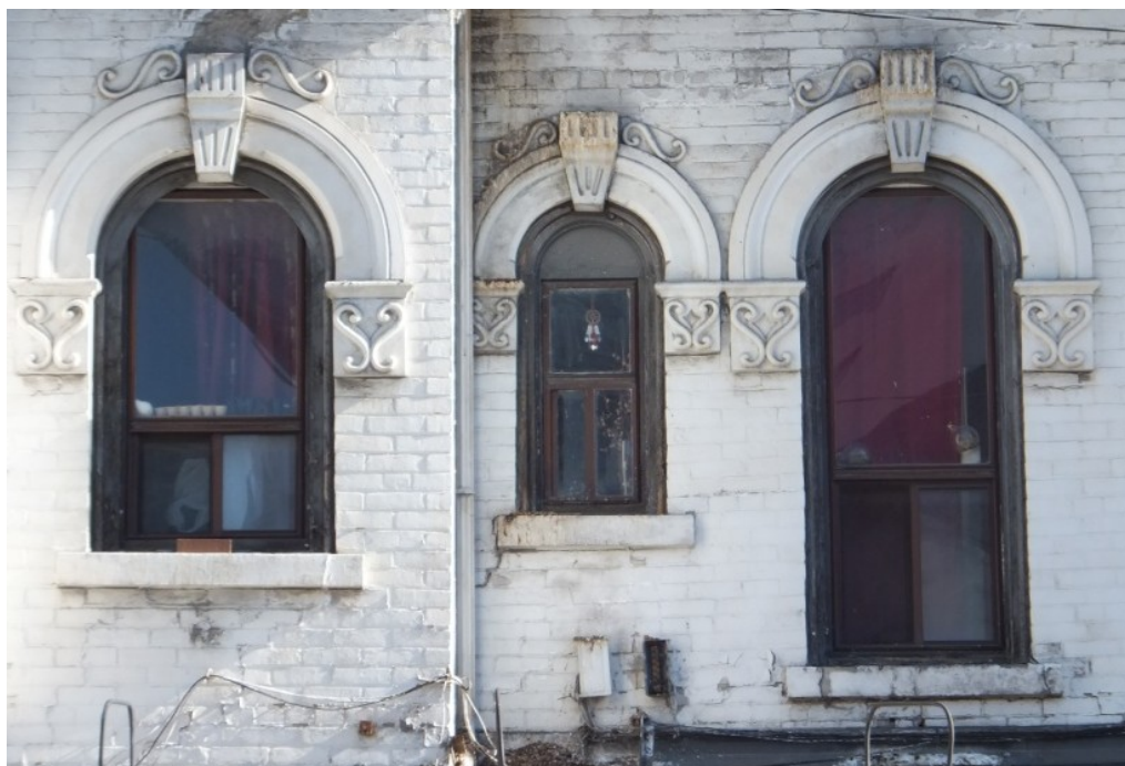
Above: window detailing; cover: William McBean Terrace, northeast corner of Church & Wellesley Streets (Heritage Preservation Services, November 2013)
