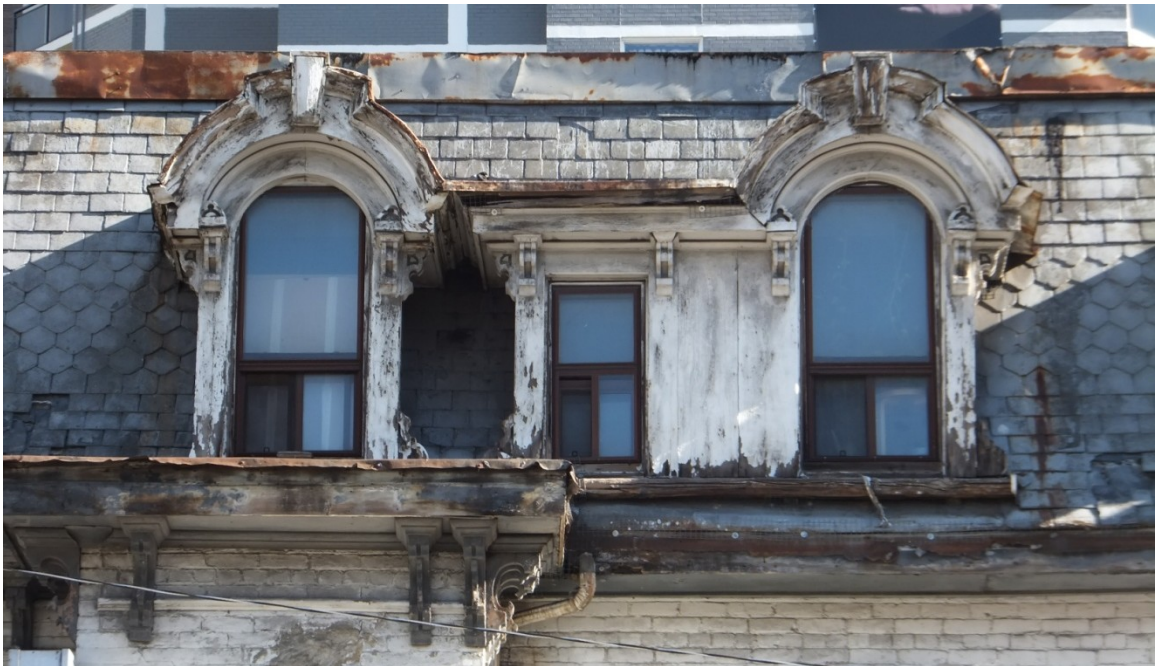
17. Current Photographs, 68 Wellesley Street East, October 2013: showing the west facade on Church Street (above), with a detail of the dormer windows, roof shingles, and bracketed cornice (below) (Heritage Preservation Services)
