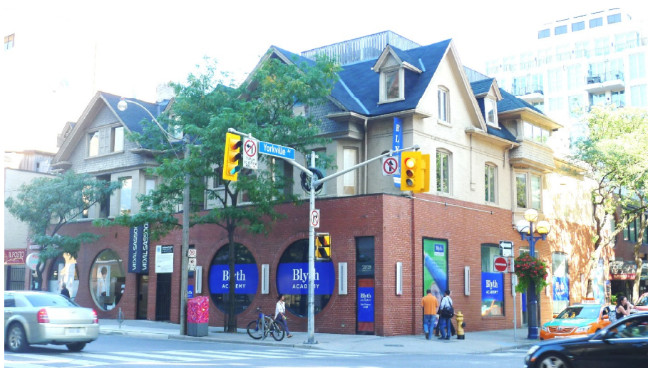
Above: York Square, West and South Facades at Avenue Road and Yorkville Avenue (HPS, 2013) Cover: York Square, South Façade on Yorkville Avenue, 1969 ( Progressive Architecture , September 1969, p 148)
