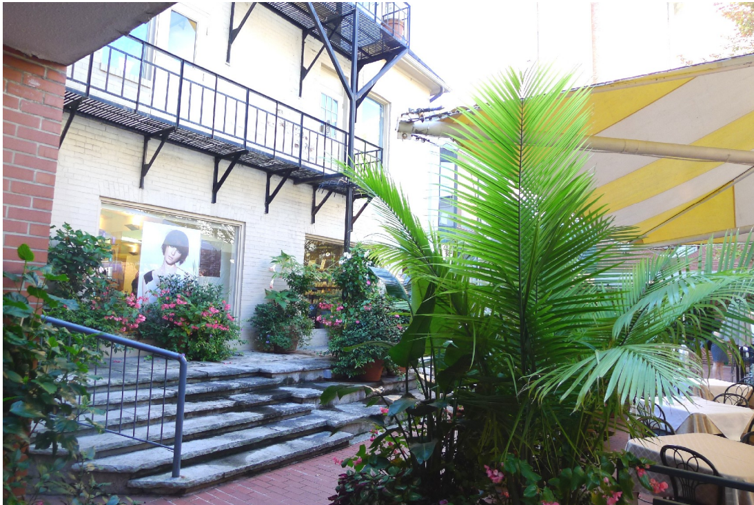
12. York Square Courtyard : Original c1900 buildings are painted and integrated into the new courtyard with new staircases and planting. ( Heritage Preservation Services, October 2013 )
