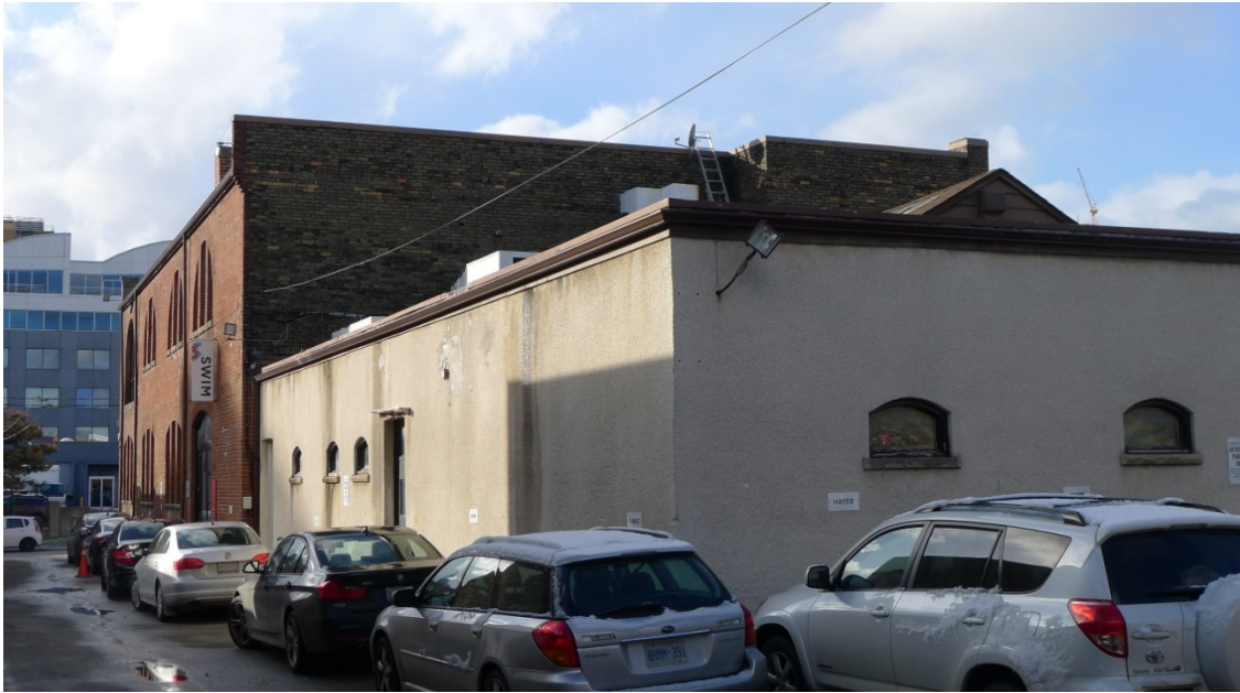
10. Current Photograph : showing the rear one-storey wing with small arched windows and stuccoed elevations. (Heritage Preservation Services, December 2013)
