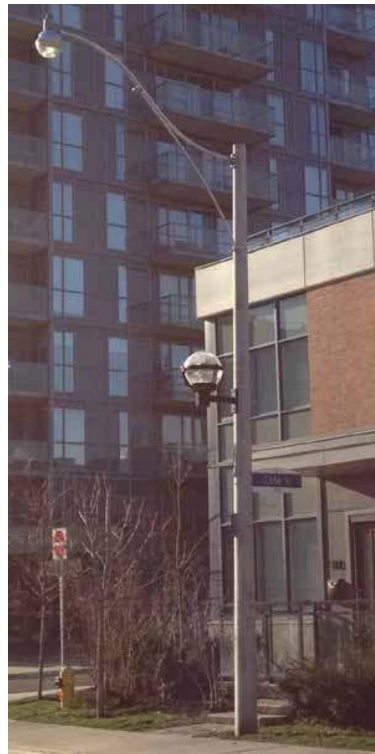
Fig. 4.10.1 Acorn street light with pedestrian lighting on same side, Regent Park, Toronto , ON
