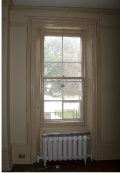
East Window(To be Removed)
