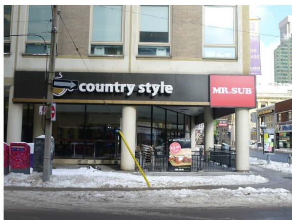
10. Corner of Yonge and St. Mary streets showing the set back of the glass façade to create an open volume at the base of the building. (Heritage Preservation Services 2014)
