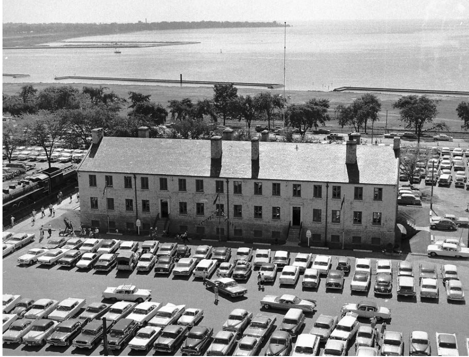
34. Archival Photographs, Officers' Quarters, 1960 : showing the north elevation of the building after it was restored as the headquarters of the Toronto Historical Board (City of Toronto Archives, Fonds 1257, Item 744)
