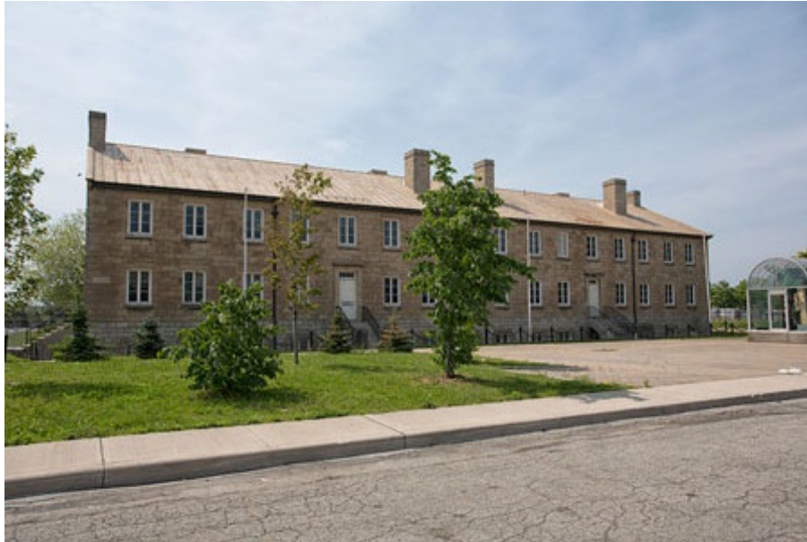
Officers' Quarters, Stanley Barracks, showing the north elevation facing Princes' Boulevard
