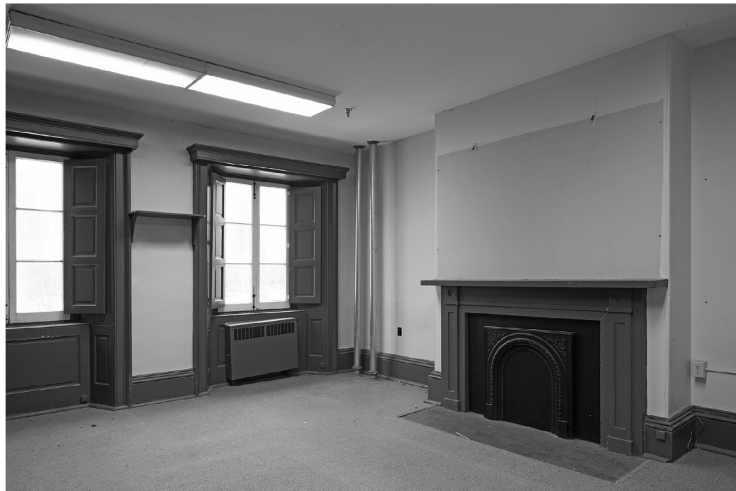
38. Interior Photographs, Officers' Quarters, 2014: showing two of the rooms with the restored original wood floors (top), woodwork (including baseboards and door and window surrounds), wood doors (some with original hardware), interior wood shutters (restored), and fireplace surrounds with mantels (Steven Evans Photography)
