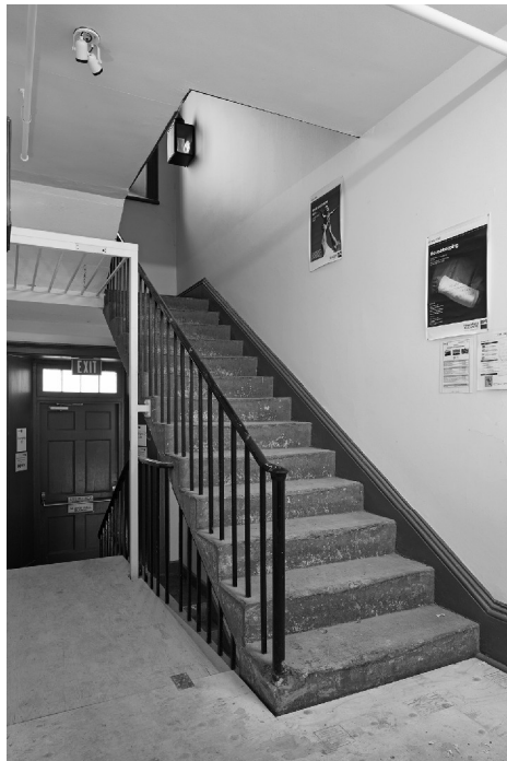
40. Interior Photographs, Officers' Quarters, 2014: showing sections of the two stone staircases with iron railings at the west end of the building that extend from the basement to the first floor (left) and from the first to the second floors (right) (Steven Evans Photography)
