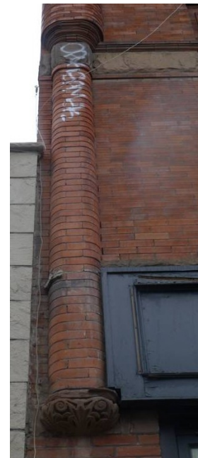
13. Dingman's Hall : showing carved stone boss (left) and curved brick colonette (right) with boss at the base, right ( Heritage Preservation Services 2014 )
