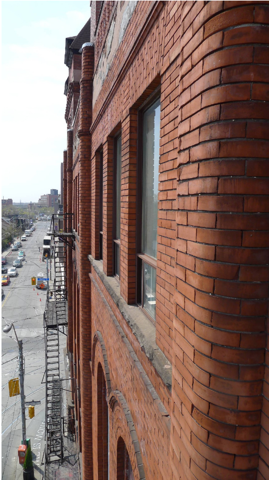
14. Dingman's Hall: at the fourth floor level Broadview façade: showing the fine surface quality, precise joints especially in the headers, profiles and curved bricks( Heritage Preservation Services 2014 )
