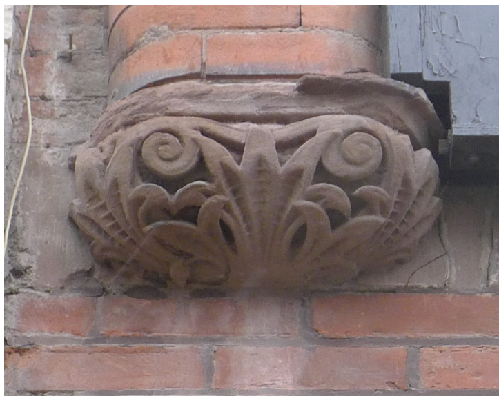
13. Dingman's Hall : showing carved stone boss (left) and curved brick colonette (right) with boss at the base, right ( Heritage Preservation Services 2014 )
