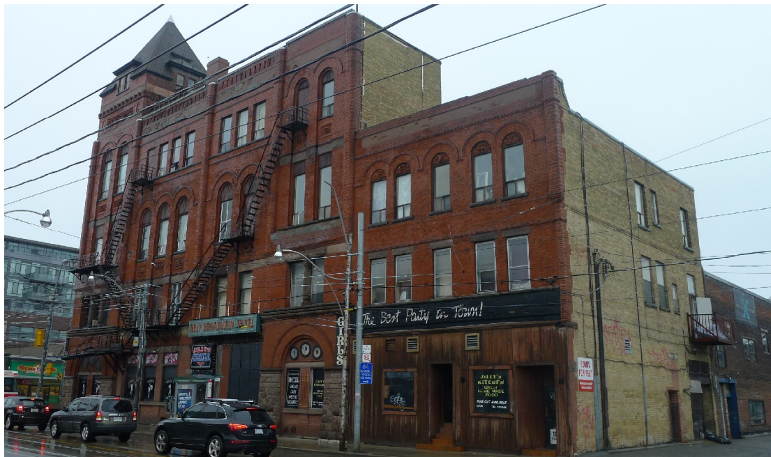
15. Dingman's Hall : showing brick details in raised moulded profiles, panels and corbelling, as well as the curved bricks used in the colonettes at the tower corners as well as cast terracotta panels, (above left) and brick colonettes in central panel above right with canted brick panels below stone sills (right) ( Heritage Preservation Services 2014 )
