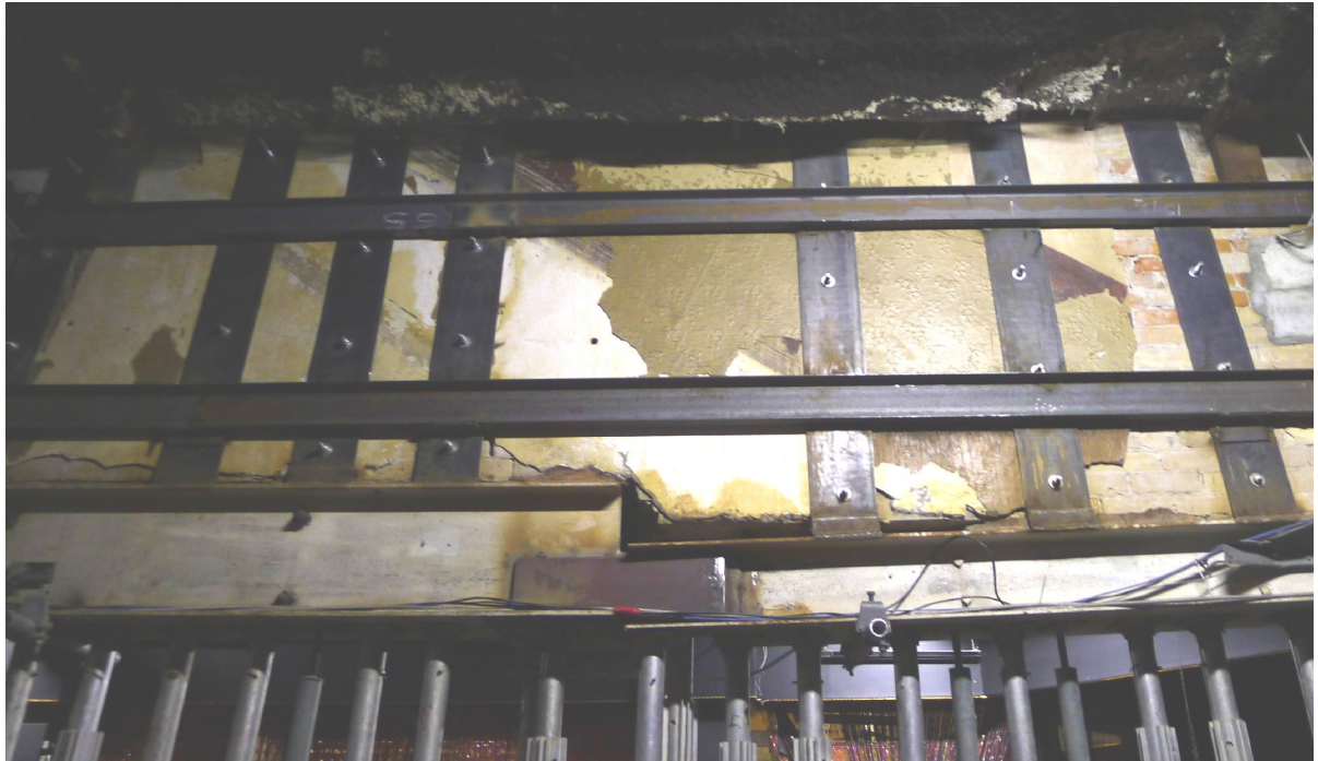
24. Dingman's Hall, former 710 Queen Street East demising wall at first floor : showing the diagonal evidence of a former staircase and possible remnants of the stair stringer. (Heritage Preservation Services 2014)
