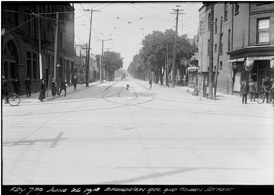
22. Broadview Avenue intersection at Queen Street East, 1918 : showing the Broadview Street façade of the hotel matching the current configuration of the arched openings without any doors or entrances and with matching sill height of the windows. (City of Toronto Archives, Fonds200, Series 372, Subseries 58, Item 750, provided by ERA Architects Inc.)
