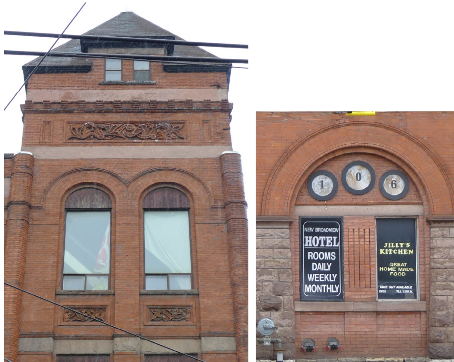
15. Dingman's Hall : showing brick details in raised moulded profiles, panels and corbelling, as well as the curved bricks used in the colonettes at the tower corners as well as cast terracotta panels, (above left) and brick colonettes in central panel above right with canted brick panels below stone sills (right) ( Heritage Preservation Services 2014 )
