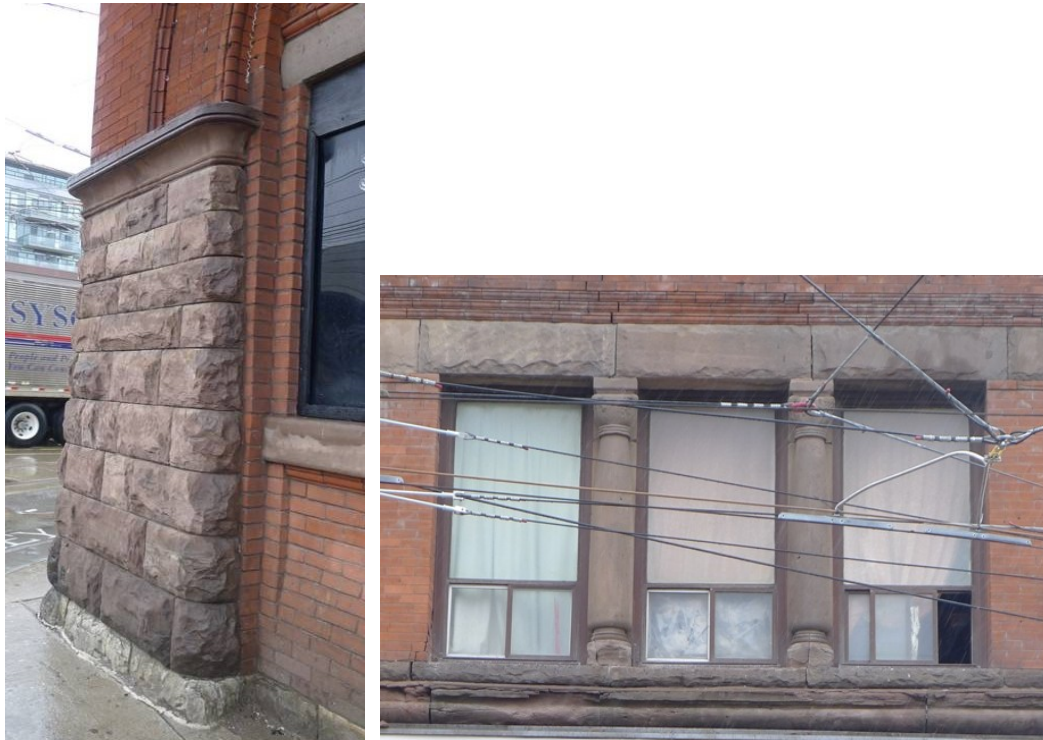
12. Dingman's Hall : showing stone details at the base of tower rough hewn blocks and smooth covered impost with linear carving. Note the canted bricks below the window sill (above left) showing carved stone columns, rough hewn lintels and sill with stone belt course below (above right) ( Heritage Preservation Services 2014 )
