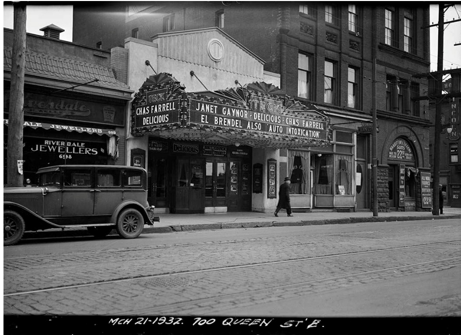
23. "Teck Theatre" 1932 : showing the Broadview Hotel with shop front at left, the door leading that originally lead to offices and public halls at 710 Queen Street East and what might have been the entrance to the bank at 712 Queen Street East. (City of Toronto Archives, Fonds 1231, Item 641 provided by ERA Architects Inc.)
