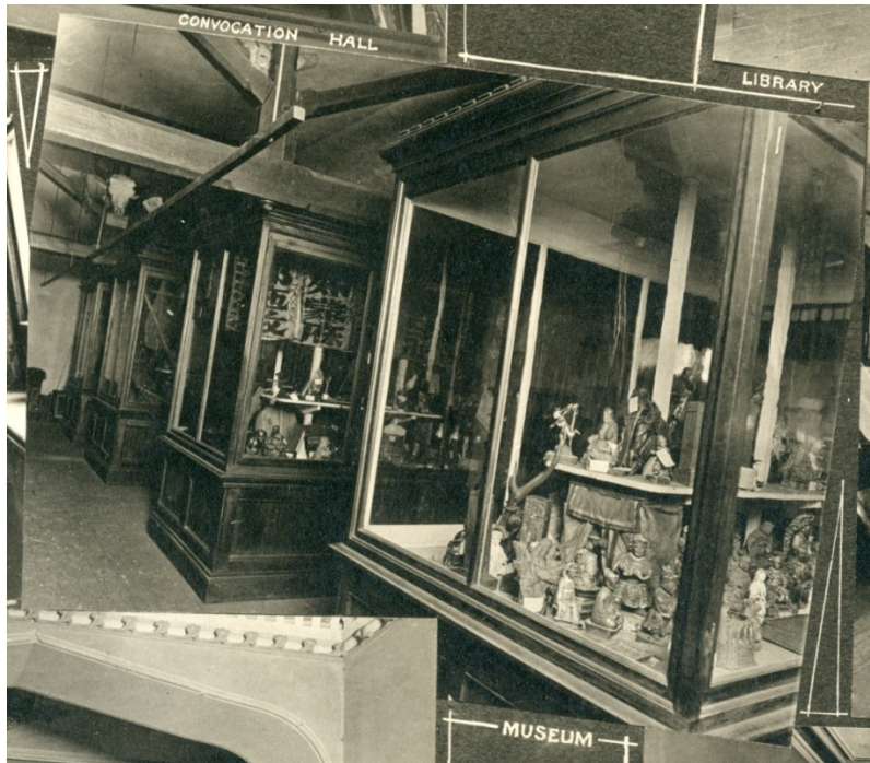
32. Knox College, Museum, Second Floor : showing the museum space as originally occupied and the exposed wooden trusses ( Heritage Preservation Services, May 2014 )
