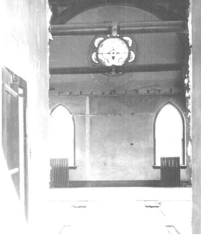
28. Knox College, main lecture hall : showing the lecture hall subdivided for medical and laboratory uses with a second floor level and shorter lancet windows. Note circular tie beams still present ( Connaught Laboratory Archives Acc0131, 1943)
