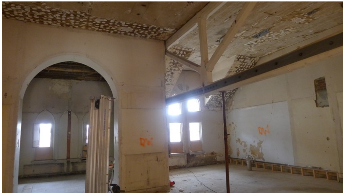
33. Knox College, Museum, Second Floor : showing the museum space with the smaller room within the tower walls and the exposed wooden trusses. Note the former arched windows
