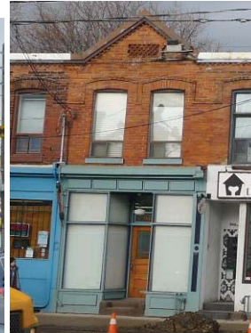
944 Queen Street East
