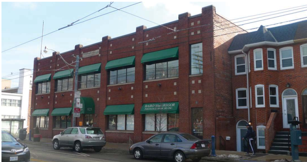
South Side, Block 1, 825 (Empire Mills) and 819-817 Queen Street East
