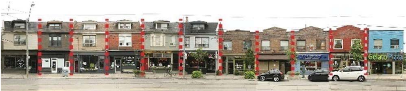
Queen Street East (Caroline Avenue to Winnifred Avenue)
