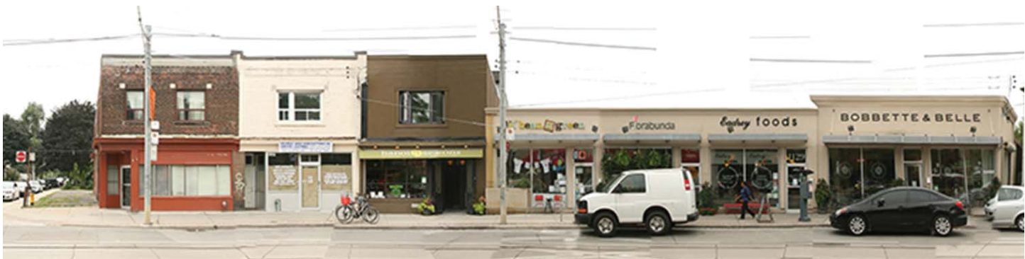
Queen Street East (Larchmount Avenue to Caroline Avenue)
