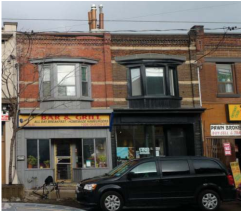
North Side, Block 6 1026-8 Queen St East
