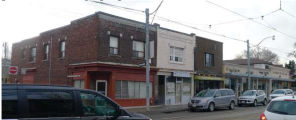
South Side, Block 10, 1139-1121 Queen Street East
