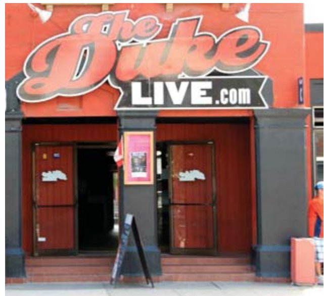
1225-1227 Queen Street East
