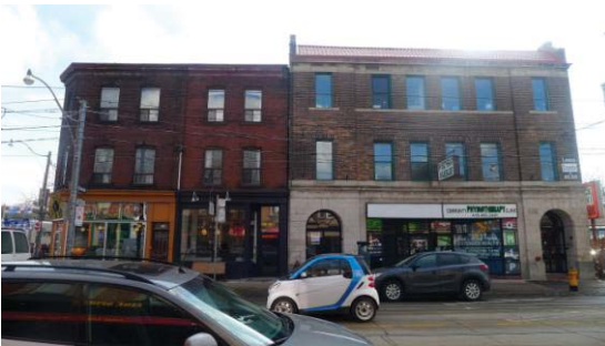
South Side, Block 4, 909-915 Queen Street East
