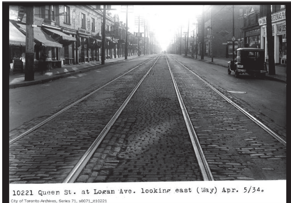
Queen Street East at Logan looking east, April 1934. The block at 922-926 Queen Street East (north side, Block 3) appears on the left hand side with its semi-circular parapet. 909-911 Queen Street East (south side) appears on the right in the distance. Immediately at the right is 889-893 Queen Street East (south side, block 3). (City of Toronto Archives, Fonds 16, Series 71)
