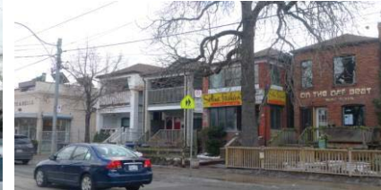
1119-1113 Queen Street East
