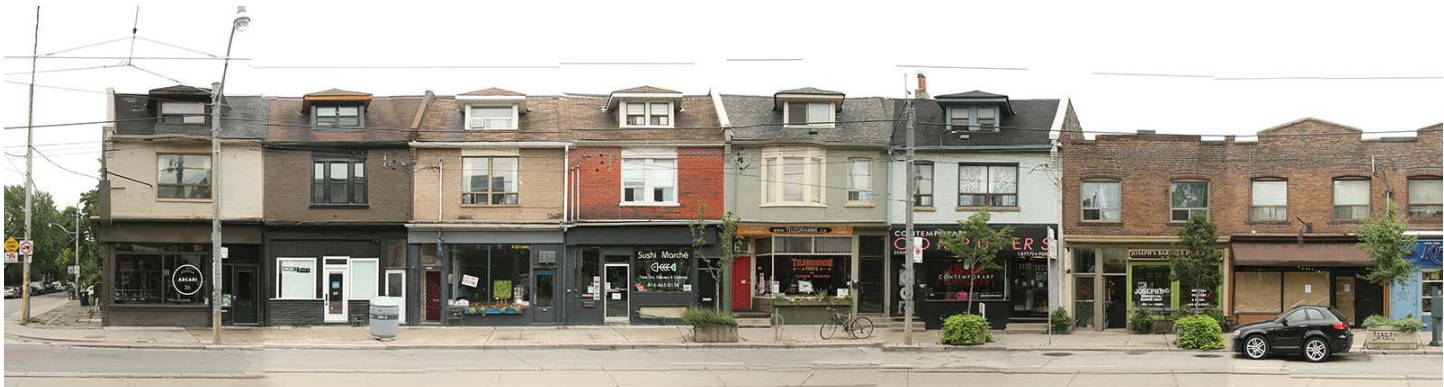
Queen Street East (Caroline Avenue to Winnifred Avenue)
