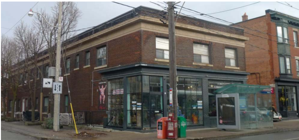
North Side, Block 8, 1100-1112 Queen St East
