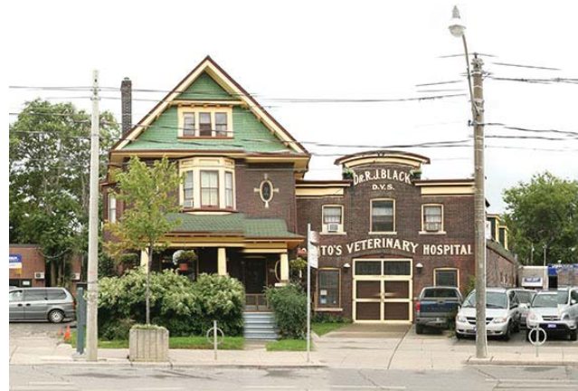
923 Queen Street East
