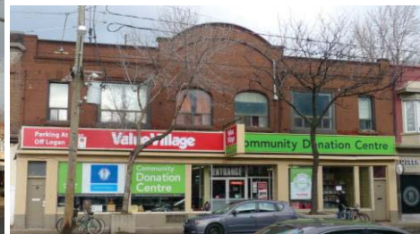
922-926 Queen Street East
