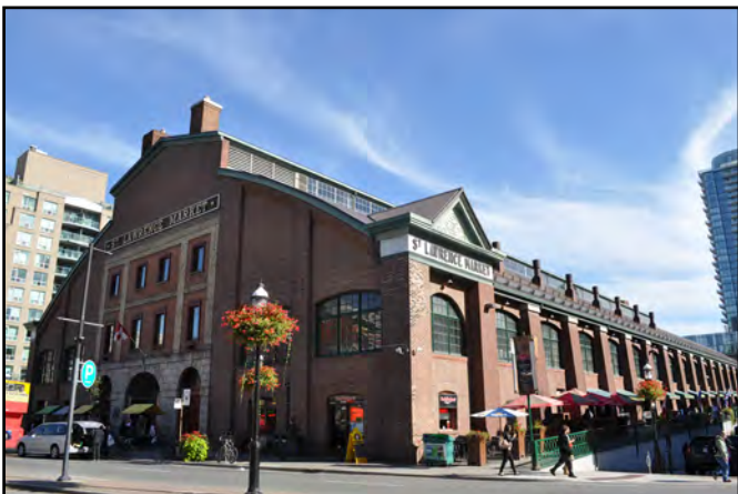
Figure 18: South St. Lawrence Market
