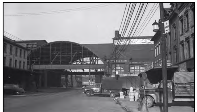
Figure 4: Demolition of the St. Lawrence Market's Front Street canopy, 1952. Virtual Reference Library, Toronto Public Library.
