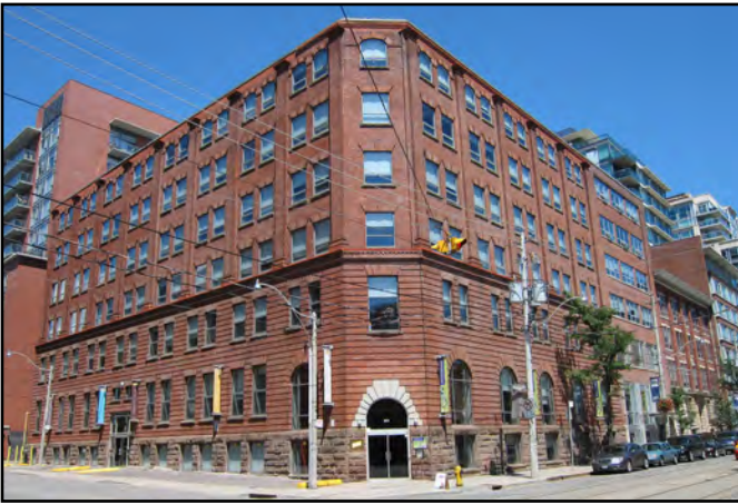
Figure 13: 204 King Street East, Industrial building typology
