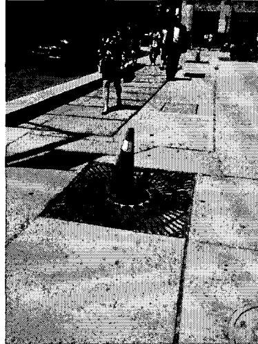
Unsafe sidewalk conditions on York Street.
