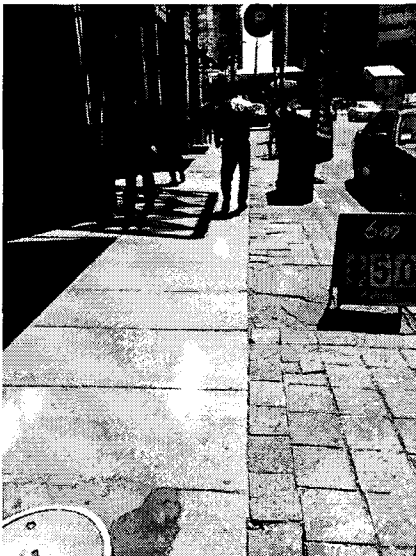
Unsafe sidewalk conditions on York Street.
