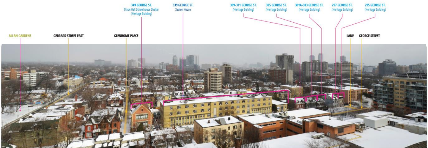
Aerial View Looking Southeast
