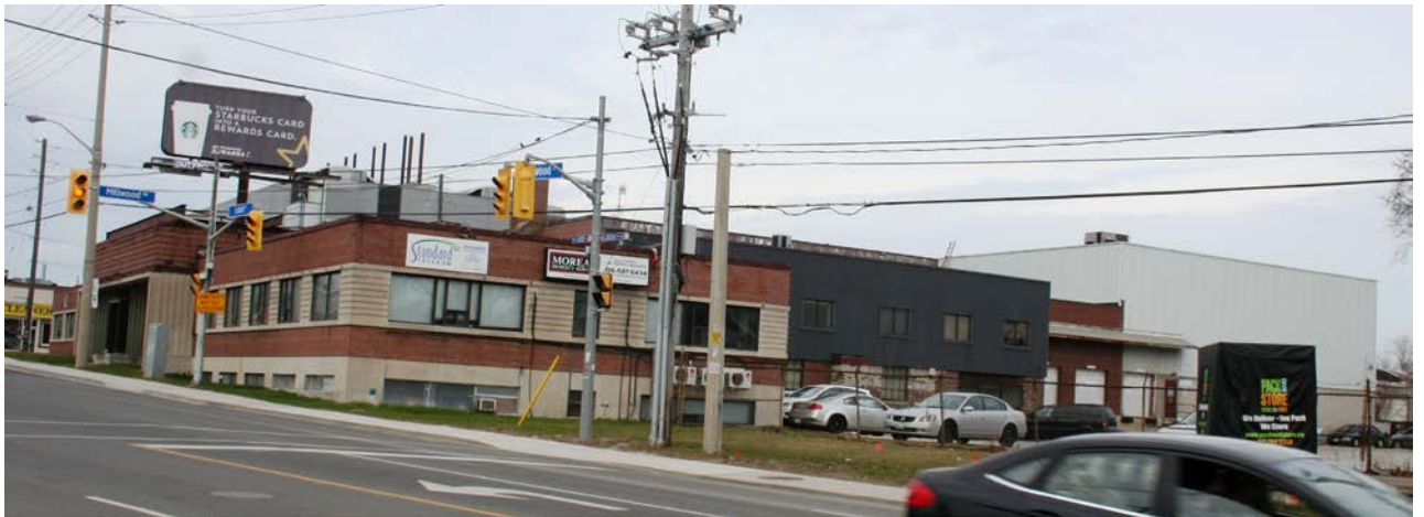
19. Sheridan Equipment Company Ltd., south-east elevations: showing the extensions (clad in white metal) and the second storey addition (clad in black aluminum siding). ( Heritage Preservation Services, 2015 )
