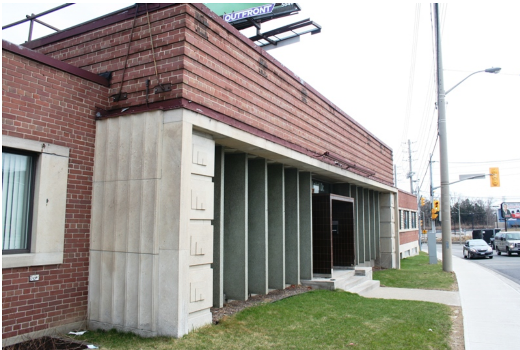
26. Sheridan Equipment Co. Ltd. : showing the main entry and showroom with the concrete frame, C-channels in the façade alternating with floor-to-ceiling glazing, cast-stone decorative elements and brick striations. Note the tile framed entry portal, greenish tone of the c-channels and the traditional "fluting" of the end side panels. ( Heritage Preservation Services, 2015 )
