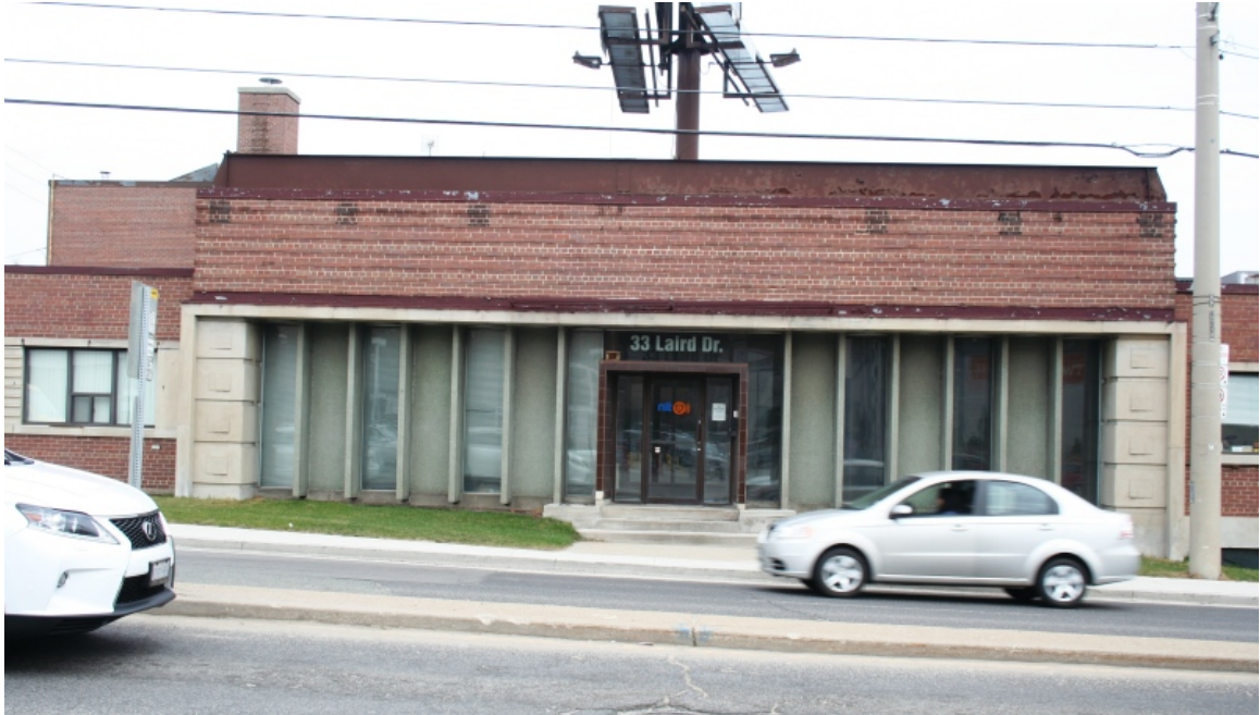
25. Sheridan Equipment Co. Ltd. : showing the main entry and showroom. ( Heritage Preservation Services, 2015 )
