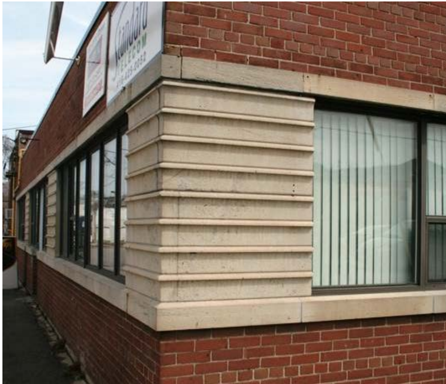
28. Sheridan Equipment Co. Ltd. : showing the Art-Deco style cast-stone panels used on the side office/stockroom wings. ( Heritage Preservation Services, 2015 )
