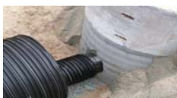
Oversized pipes can be used to temporarily store peak sewage flows for controlled release, reducing the frequency and severity of excessive hydraulic loading to the pipes.
