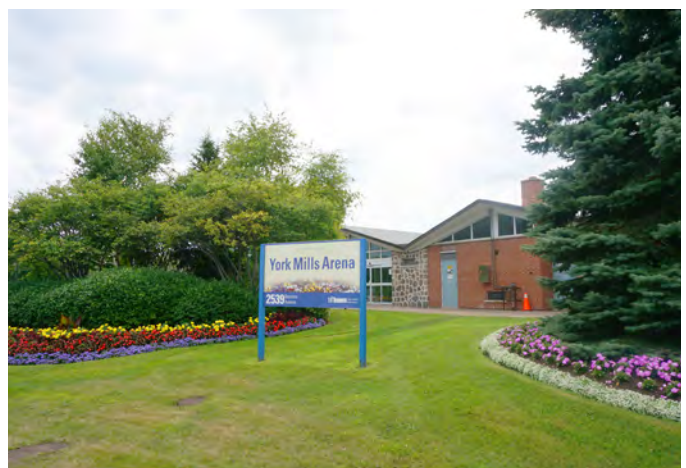
Figure 20: York Mills Arena
