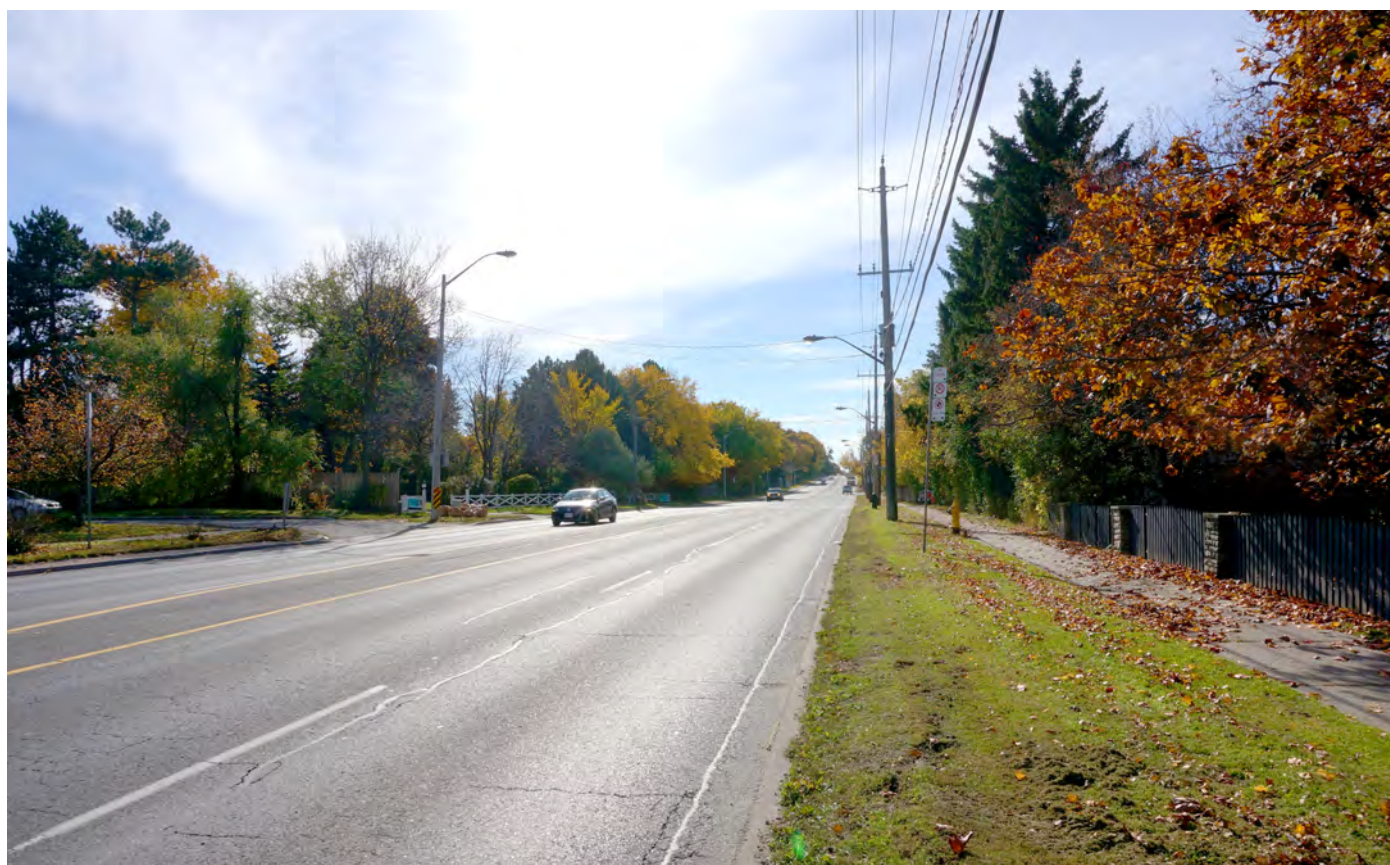
Figure 1: Bayview Avenue looking South from York Road
