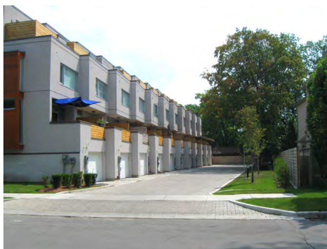
Figure 35: An example of servicing and utilities located at the rear of the townhouse development
