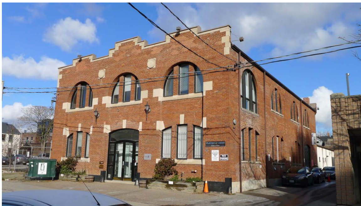
Above: Principal (west) and side (south) elevations of the Christie, Brown & Co. Stables (Heritage Preservation Services, December 2013)
