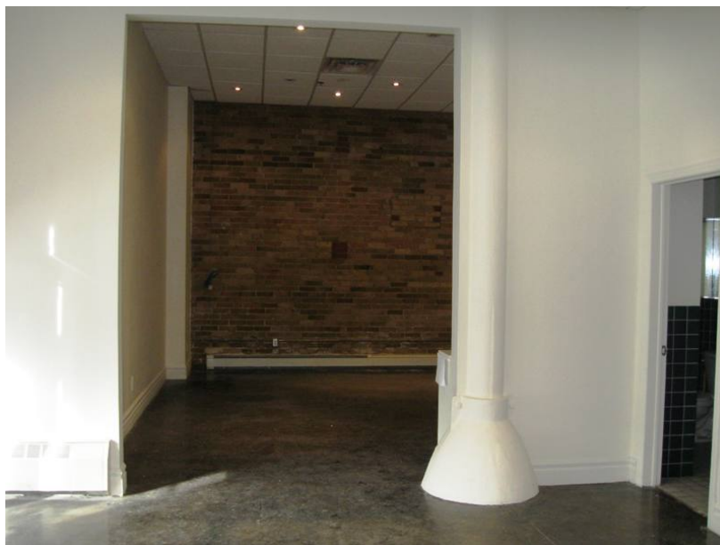
19. Carriage house interior : showing remaining steel column with protective bollard that lined the carriage entry way. ( Heritage Preservation Services, January 2014 )
