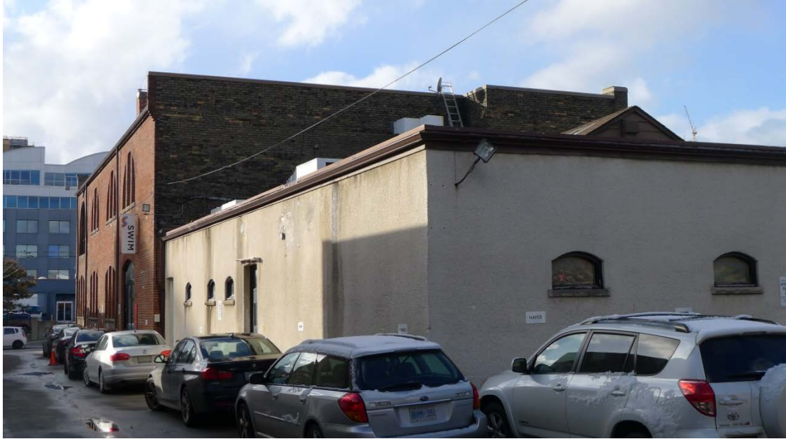
10. South and West Elevations : showing the rear one-storey wing with small arched windows for the horses' stalls and stuccoed elevations. ( Heritage Preservation Services, December 2013 )
