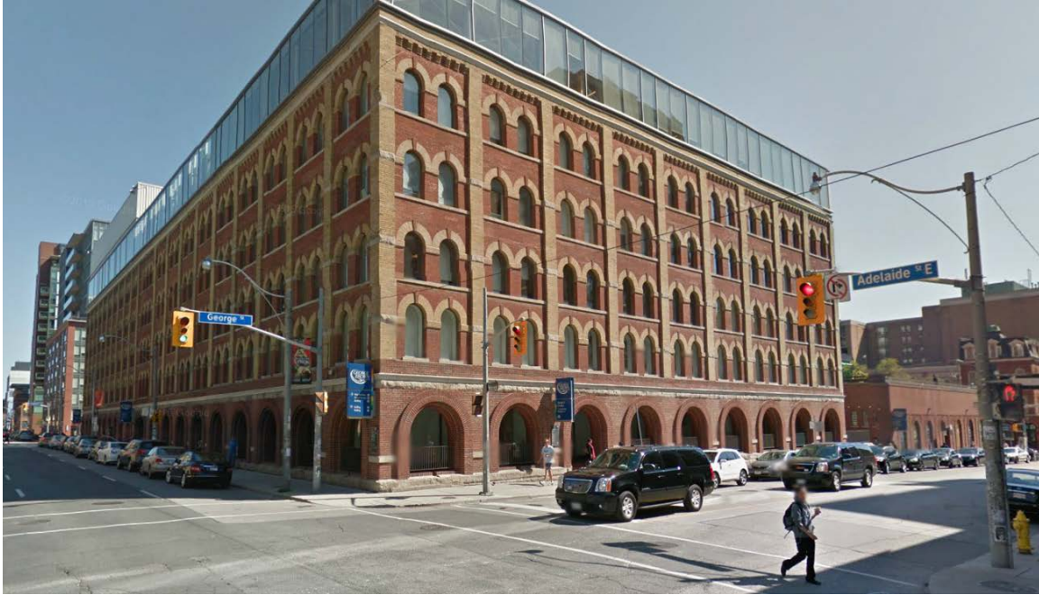
12. Biscuit Manufactory of Messrs.Christie, Brown & Co., now George Brown College : showing the full height pilasters, round-headed windows. Note the base has been altered and the pediment has been removed .
