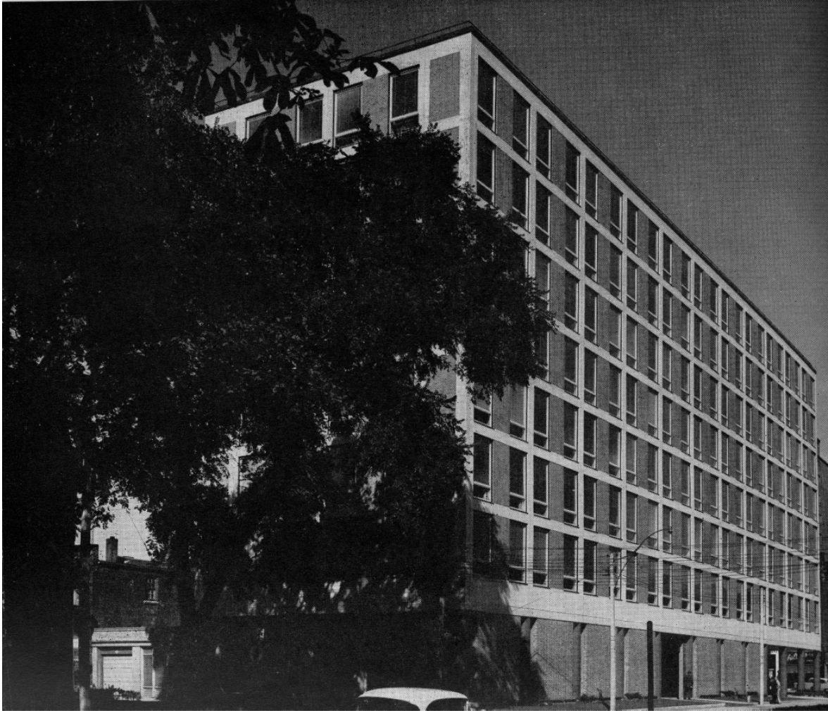
c. 1959 view looking east
