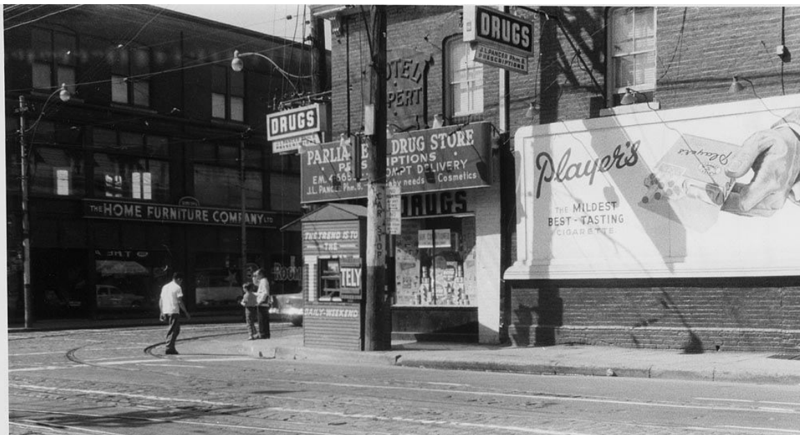
18. North West corner of Parliament and Queen Street E, August 1959 : showing the north elevation of HFCC after the cornice has been removed. (City of Toronto Archives, Series 372, Item 0376)
