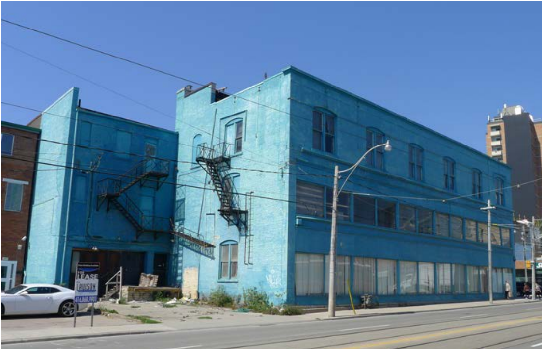
17. HFCC, south and east elevations facing Parliament Street : showing the east elevations with the window transoms covered over with boards and the south elevations indicating the extent of the original 1907 and the larger extension of 1925-6 (left of photo). (HPS 2015)
