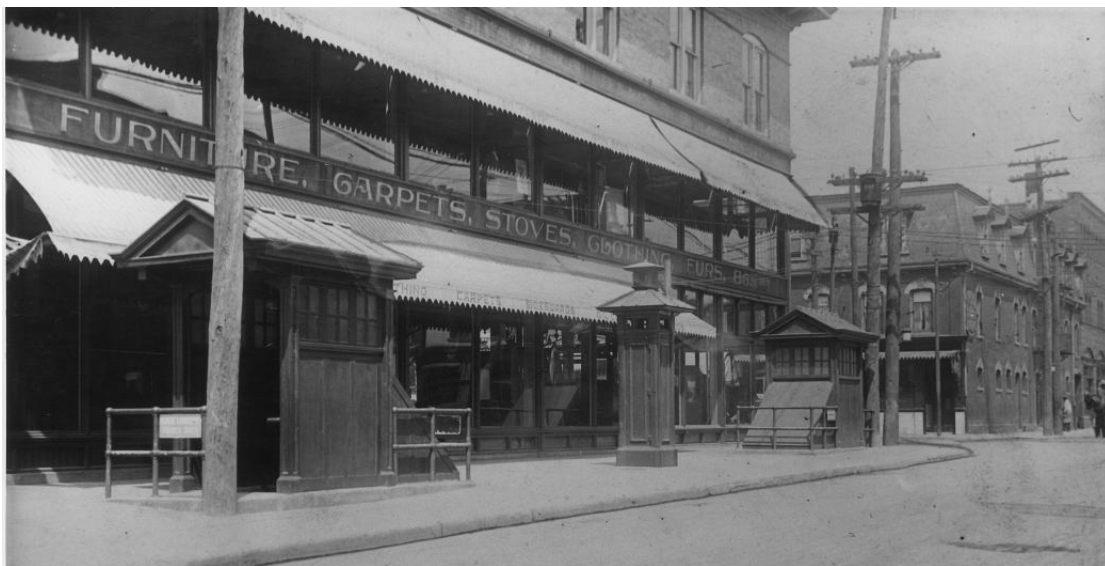
14. HFCC, east elevation on Parliament Street , 1913 (detail) : showing the awnings, a glimpse of the extent and substance of the overhanging cornice and the late Victorian context across the road. ( City of Toronto Archives, Fonds 1244, Item 7308 )
