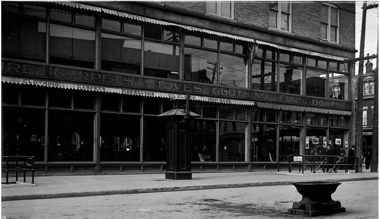
13. HFCC, east façade on Parliament Street , 1914 (detail) : showing the details of the glazing on the two lower floors, with the large glazing panels grouped in pairs between the minimal vertical structural supports with transom lights divided into pairs above each large pane, and the narrow paired panels at grade. At the third floor segmental arched windows contain a pair of double-hung sash. Note the brick entablature and moulding between the second and third floor and the narrow signage panel between the first and second floors. ( City of Toronto Archives, Fonds 1231, Item 1295 )
