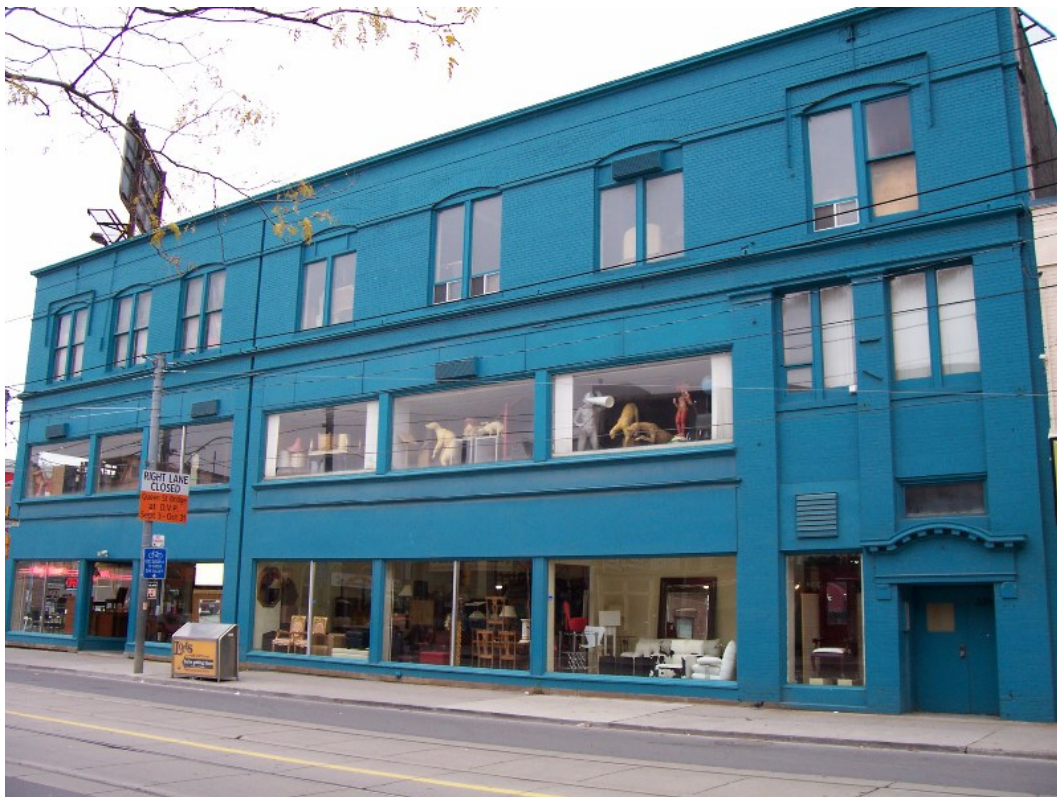
16. HFCC, north elevation on Queen Street : showing the extension with the wider bays to the west of the original store with the new entrance to the bowling club and the covering of the window transoms with board. (HPS, 2005)
