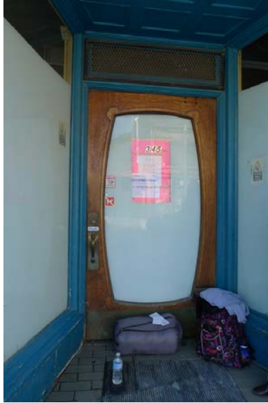
15. HFCC, Queen Street Entrance : showing the recessed glazed entrance bay, tapering in plan towards the door and the wood door with its curved glazed panel with circular corner ornaments that reveals the influence of the more organic Art Nouveau style during this period. (HPS 2015)
