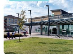
Warden Hilltop Community Centre Section 37 enhances the physical and social health of our communities by upgrading existing recreation centres and by building new facilities.
