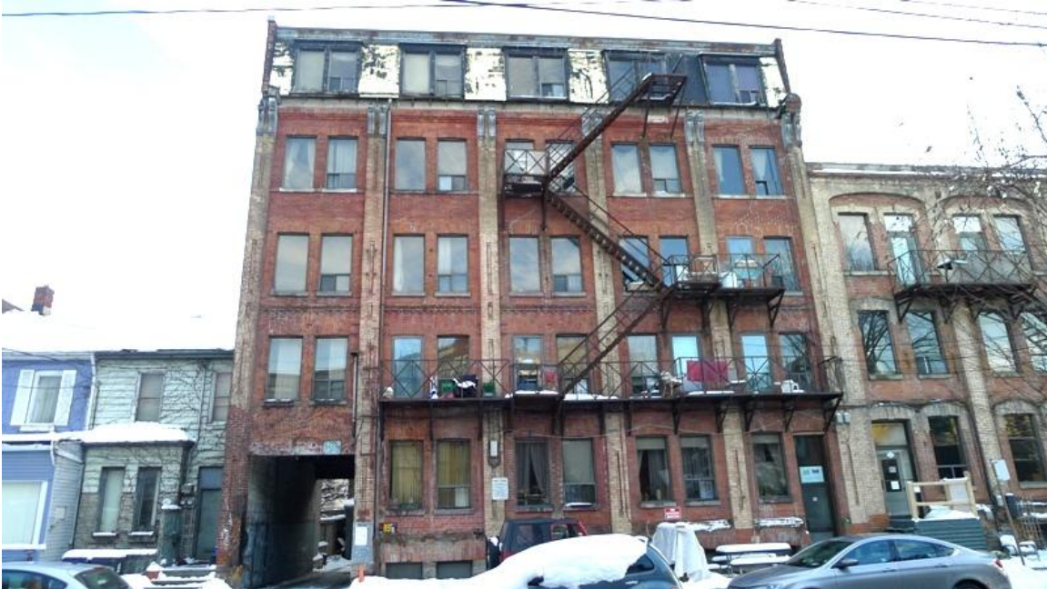
Showing the principal (north) façade of 89-91 Niagara Street, 1883-4 as illustrated in 1897 (top Toronto Board of Trade , 1897) and as photographed in 2014 (bottom, Heritage Preservation Services )
