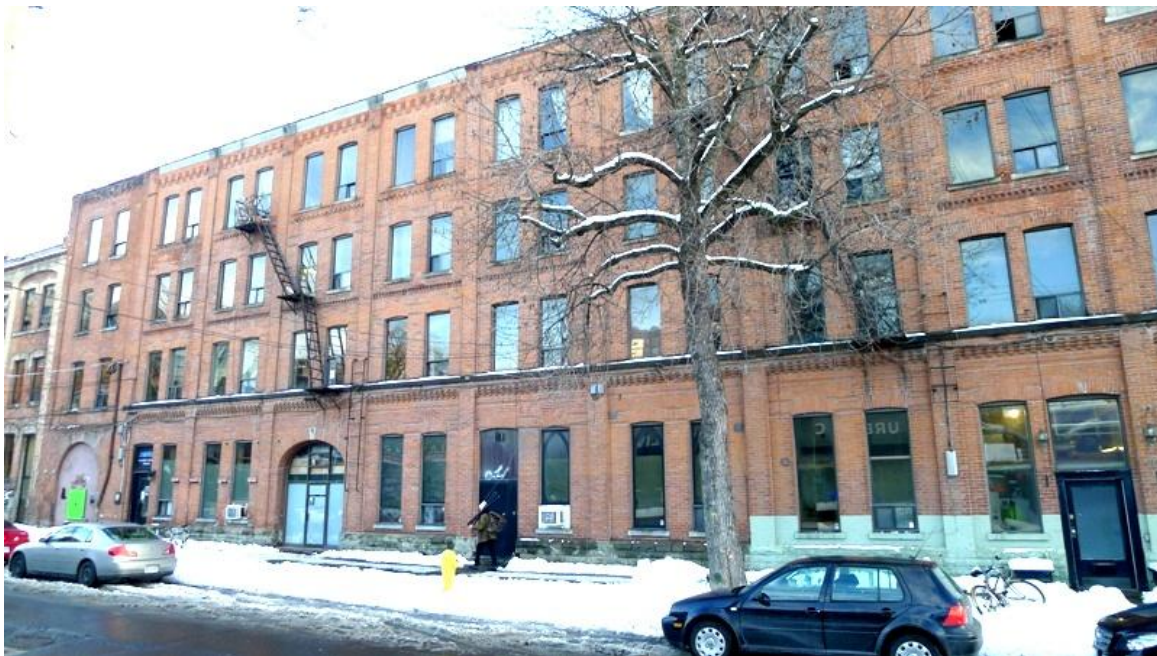
Showing the principal (north) façade of 101-107 Niagara Street, 1887 as illustrated in 1897 with the edge of 109 Niagara Street at the right (top Toronto Board of Trade , 1897) and as photographed in 2014 ( Heritage Preservation Services )
