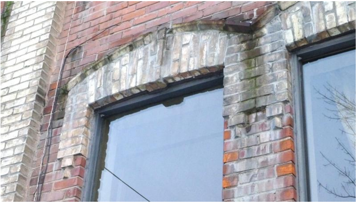
22. 95-97 Niagara Street : showing a detail view of the window hoods, keystones, projecting drip moulding and drop pendants (Heritage Preservation Services 2014)
