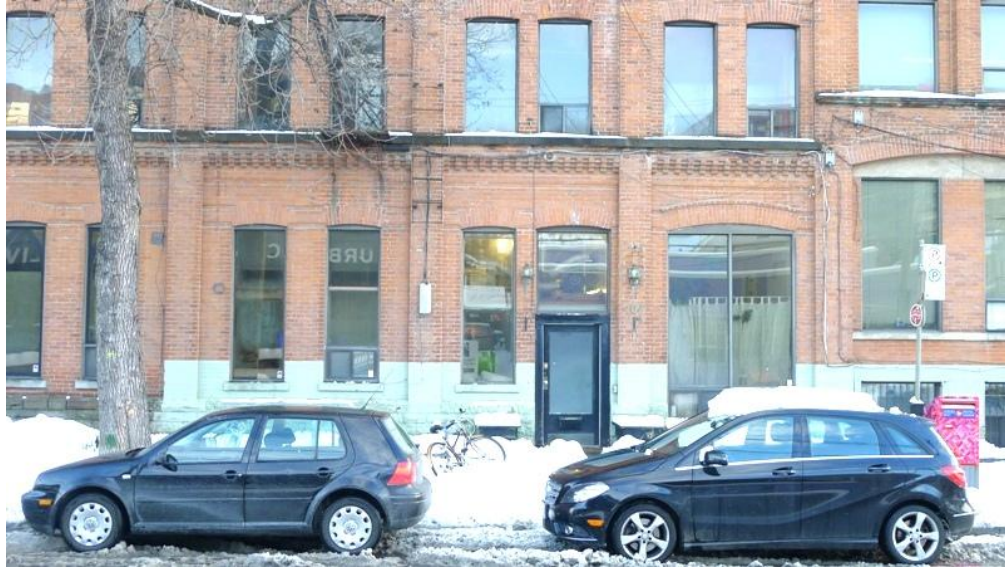
25. 101-7 Niagara Street: showing the glazed end bay which may have provided an additional passageway to the rear yard and the adjacent original doorway as well as the decorative stone belt course and brick corbels separating the first and upper level pilasters (Heritage Preservation Services 2014)
