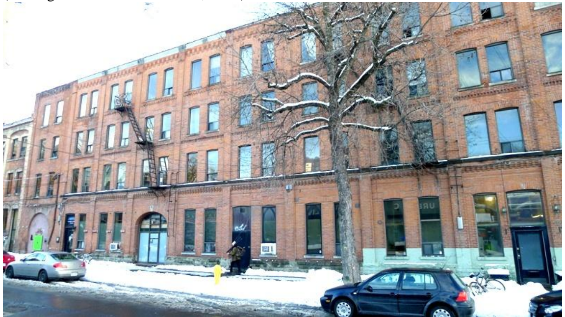
24. 101-107 Niagara Street : showing primary façade with various entrances and access points (Heritage Preservation Services 2014)
