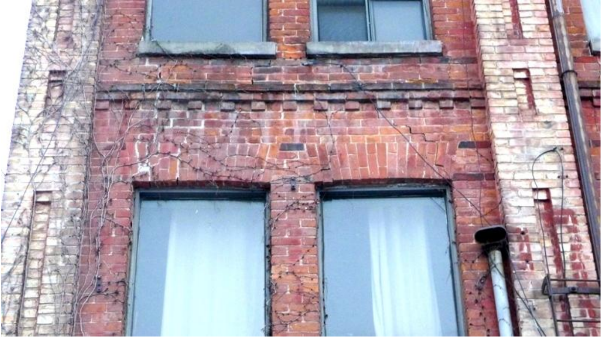
23. 89-91 Niagara Street : showing a detail view of the decorative string courses and dentil course between the floors and the relief panels in the buff brick pilasters (Heritage Preservation Services, 2014)
