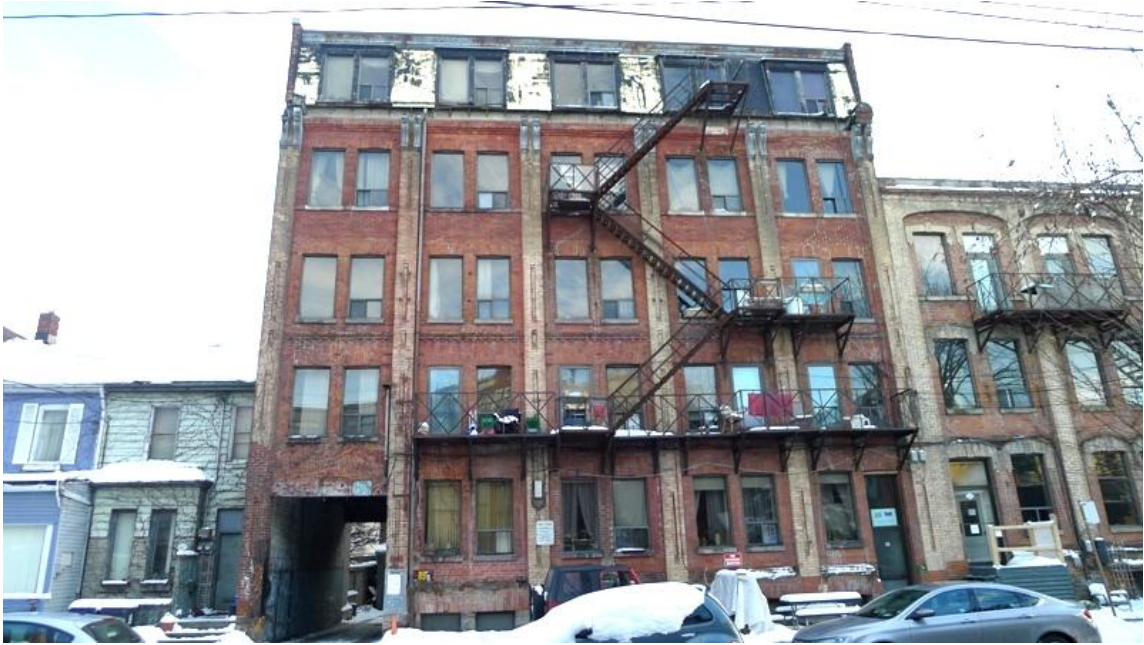
15. 89-91 Niagara Street : showing the street façade with its red brick façade, full-height buff brick pilasters, carriageway, raised basement and later mansard roof (Heritage Preservation Services 2014)
