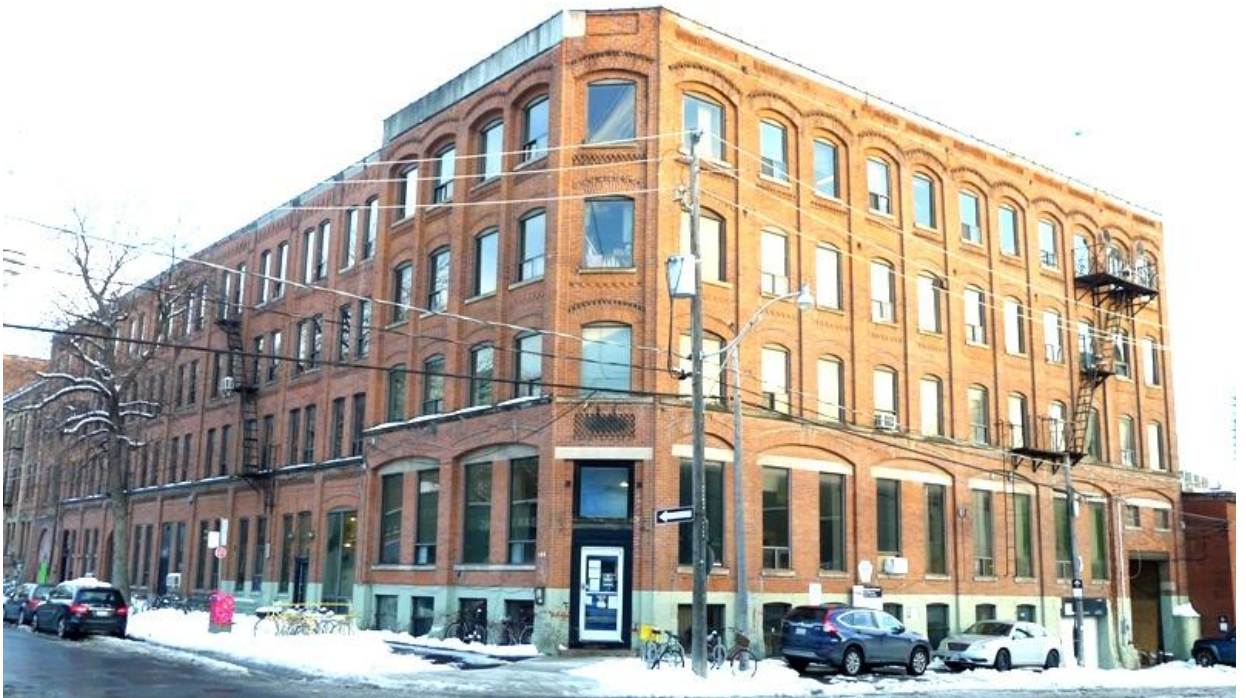
31. 109 Niagara Street : showing the decorative brick dentil courses and corbelling with the remainder of the capitals on the pilasters (Heritage Preservation Services, 2014)
