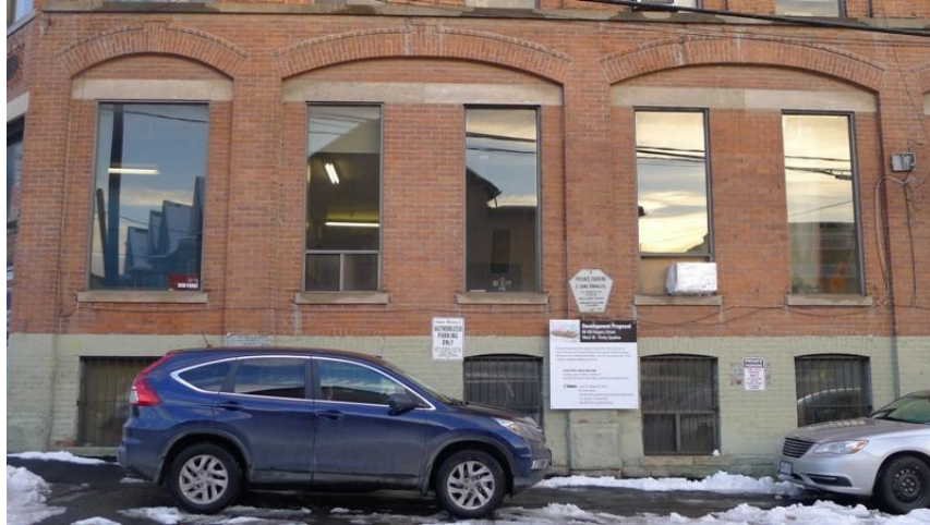
34. 109 Niagara Street : showing the first floor with the flat headed windows with the stone lintels paired with an arcade with a raised brick moulding creating a keystone and the raised basement (Heritage Preservation Services, 2014)
