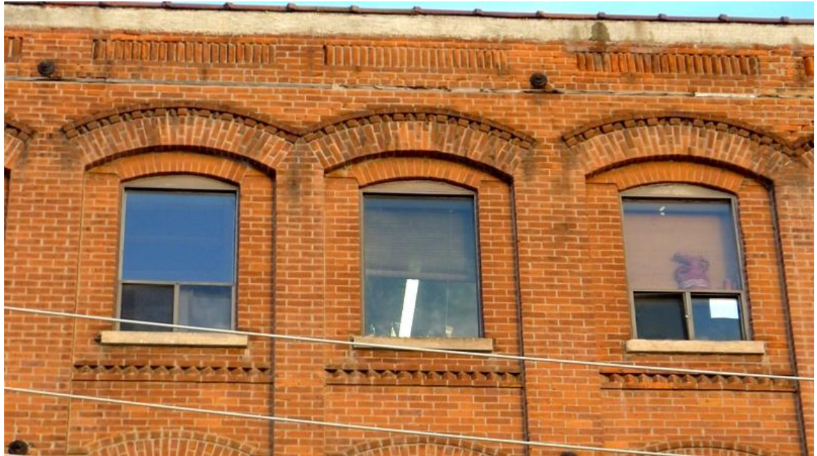
36. 109 Niagara Street : showing the upper levels arcade with the various brick details and the parapet with decorative brick panels above and stone sills (Heritage Preservation Services, 2014)
