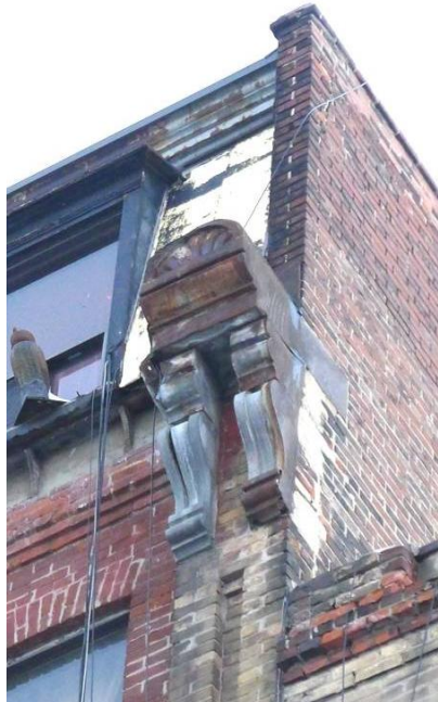
19. 89-91 Niagara Street : console brackets. (Heritage Preservation Services 2014)
