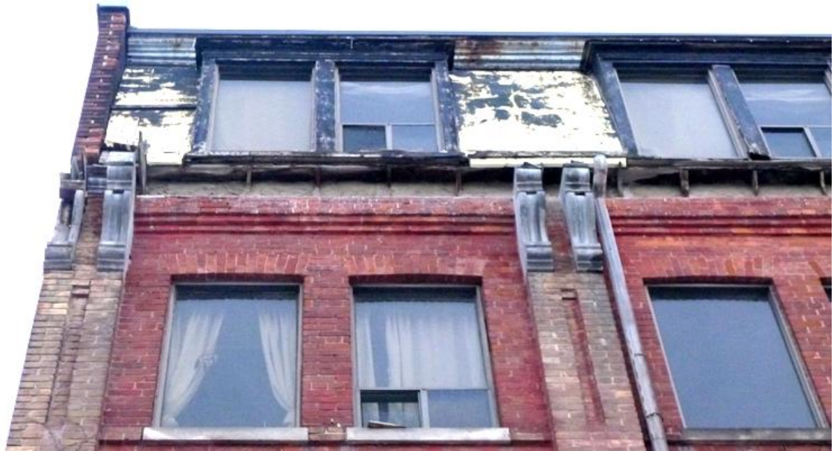
18. 95-97 Niagara Street : showing the details of the paired consoles, opening of the carriageway with its wood beam, metal tie rods and relieving brick arch above (Heritage Preservation Services, 2014)
