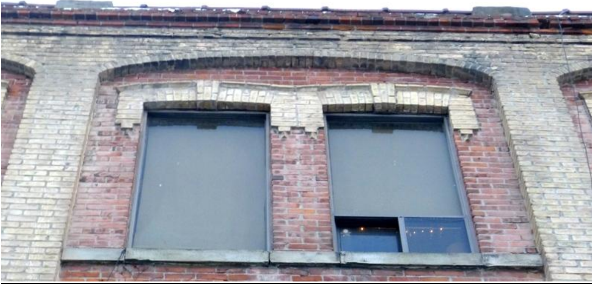
21. 95-97 Niagara Street : showing the elliptical arches and the paired window hoods, with keystones with projecting drip moulding and drop pendants at the sides (Heritage Preservation Services 2014)
