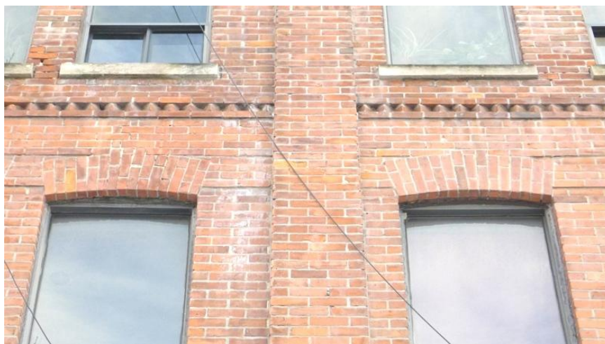
29. 101-7 Niagara Street : showing the decorative brick saw-tooth bands and the relief bands on either side of the window lintels (Heritage Preservation Services, 2014)
