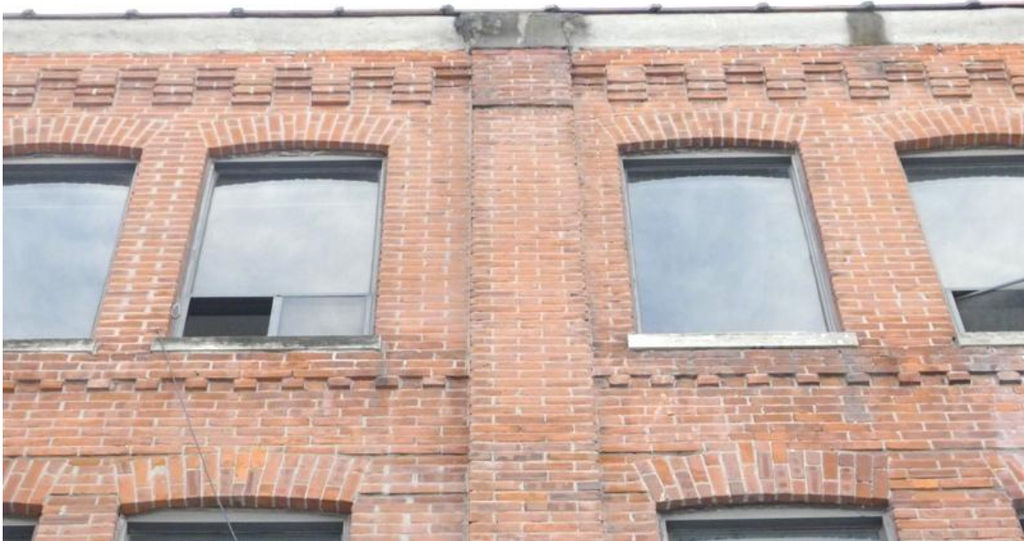
30. 101-7 Niagara Street : showing the decorative brick dentil courses and corbelling with the remainder of the capitals on the pilasters (Heritage Preservation Services, 2014)
