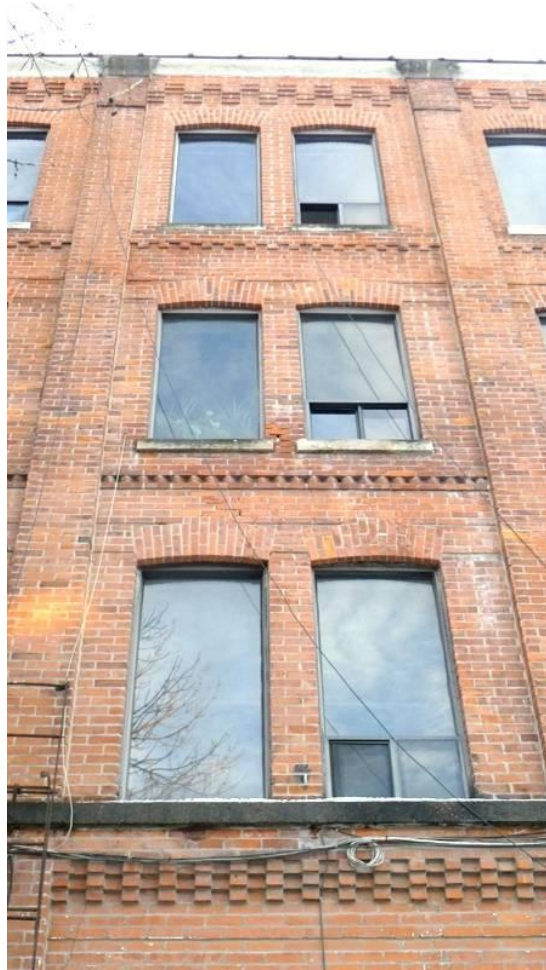
28. 101-7 Niagara Street : showing the decorative brick bands and stone belt course between each floor (Heritage Preservation Services 2014)
