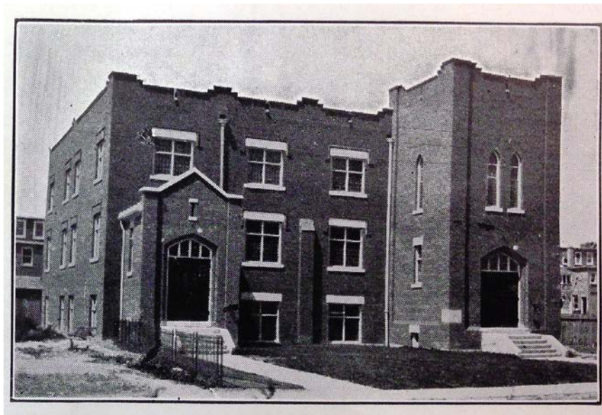
12. Jones Avenue Sunday School, East Elevation, Burke, Horwood & White, 1913: showing the church as built showing the additional tower, buttresses on the street elevation and flat roof with crenellations (not included in the original scheme) and a modified version of the entry porch, the same design for the windows (Temple Baptist Church, 1937, p 7)
