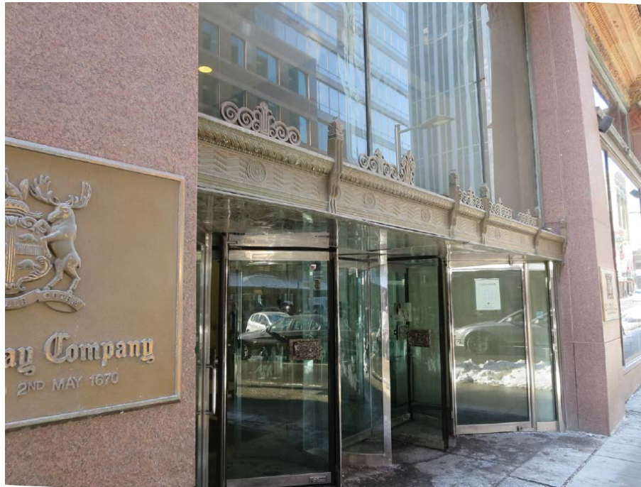
176 Yonge Street showing second bay of building on Richmond Street with non-original revolving doors, etched glass transom, and decorative bronze cornice.
