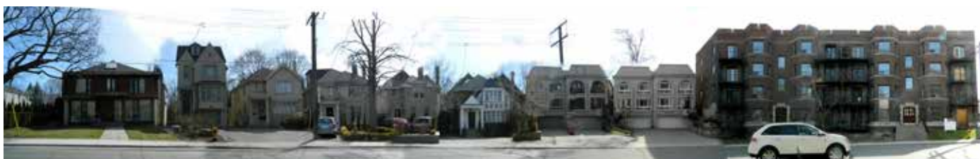
Coulson Avenue to approximately Strathearn Blvd.
