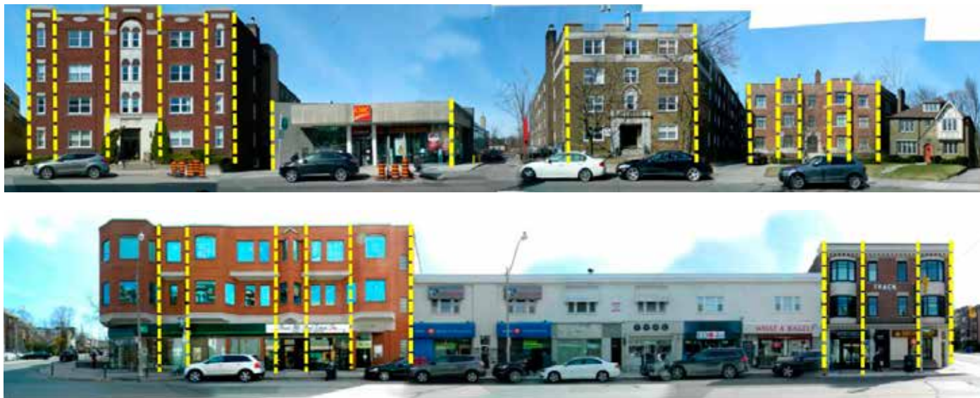
Sample of building facades and details within the Study Area
