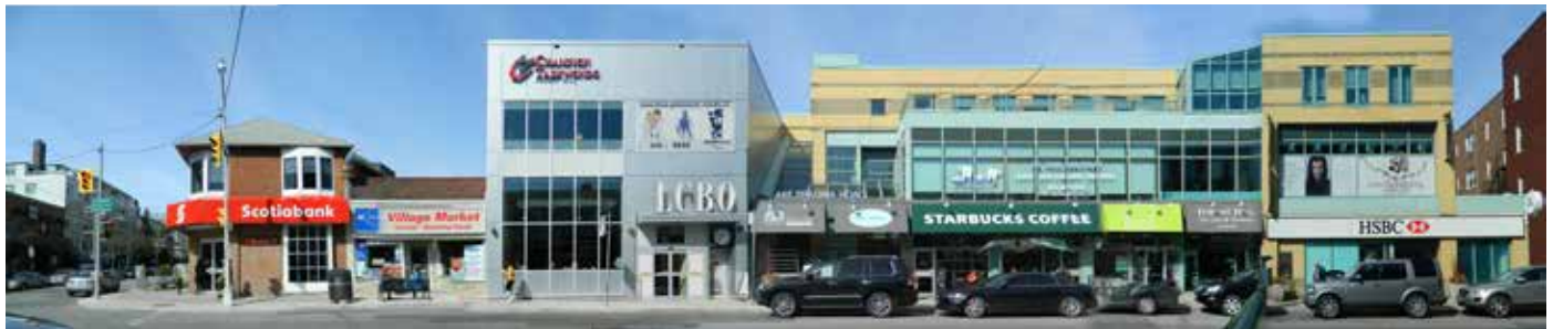
Lonsdale Avenue to approximately Thelma Avenue
