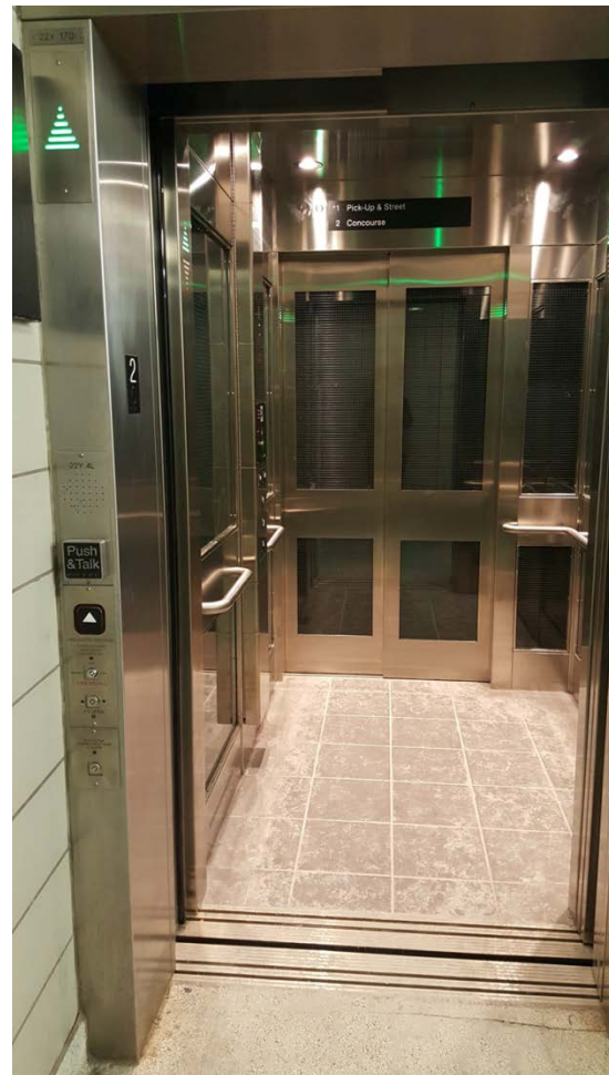
Figure 1: Modernized Elevator at Finch Station
