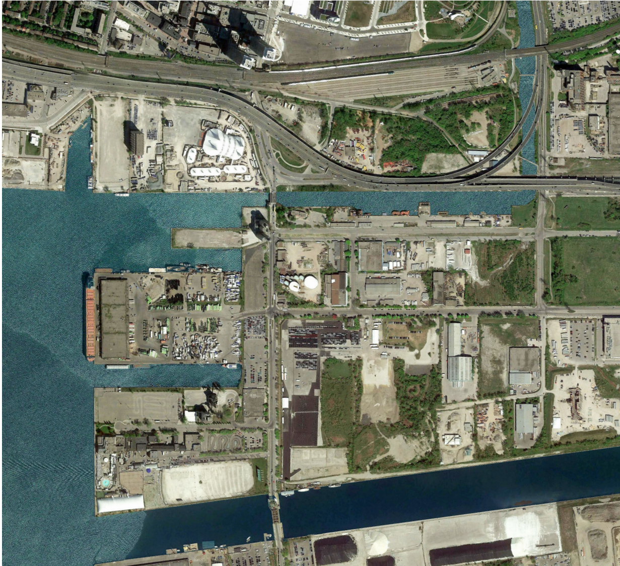
Figure 4 Aerial View of Existing Conditions
