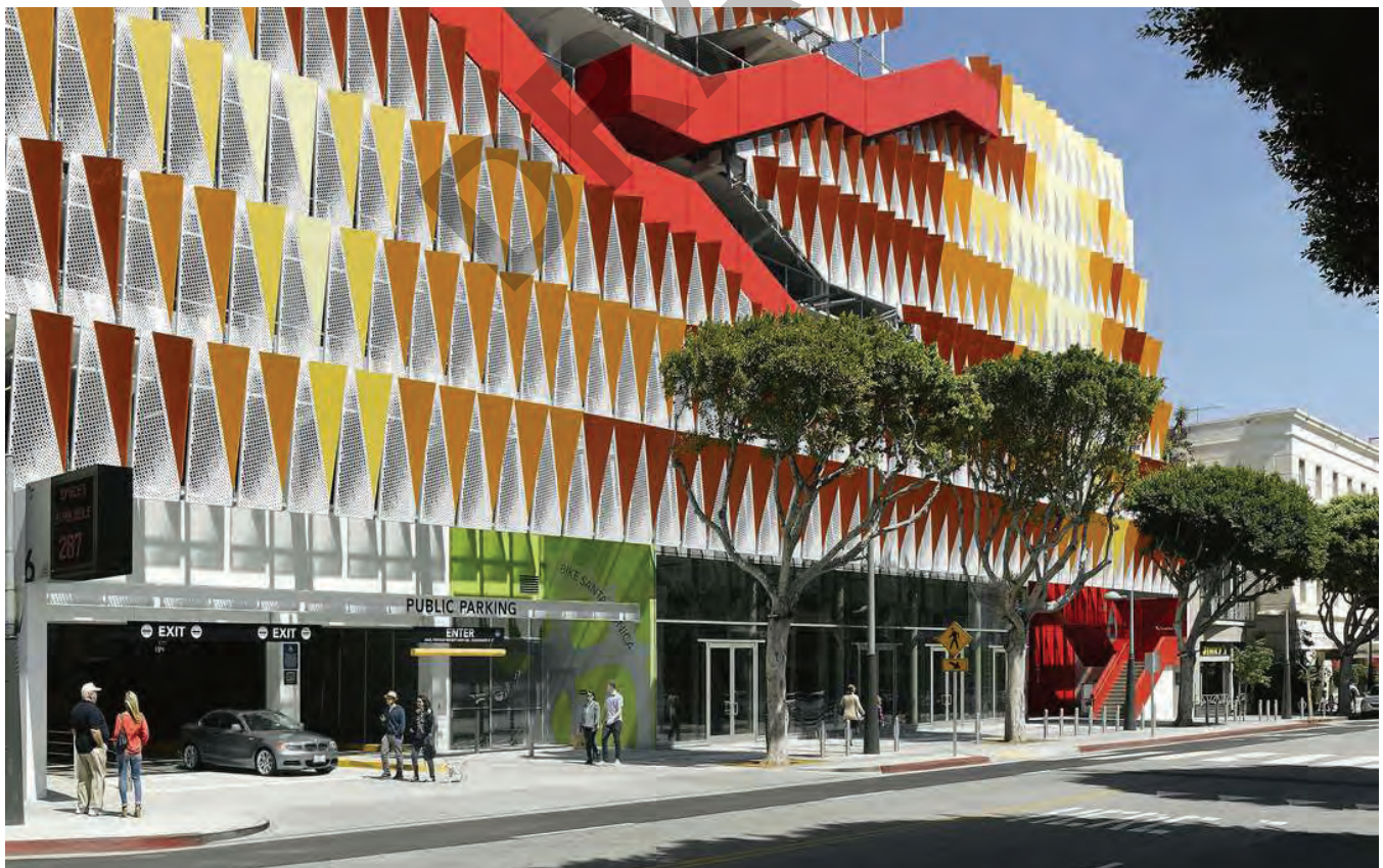
Parking structures should have the qualities of good urban buildings and provide a positive contribution to place making and identity (Santa Monica, CA. c. Behnisch Architekten)
