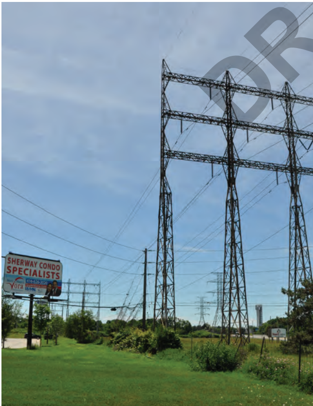
Hydro Towers at the north end of the Study Area
