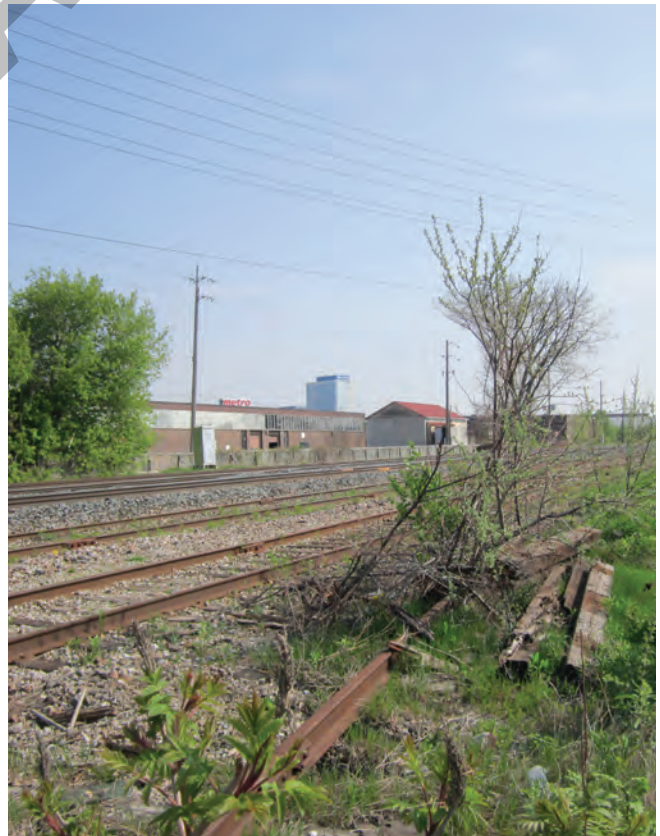
CN Rail Line at the northern edge of the Study Area
