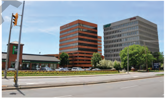
Existing office buildings along Evans Avenue
